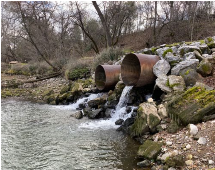
Figure 7. Existing Jenny Creek Culvert Discharge
