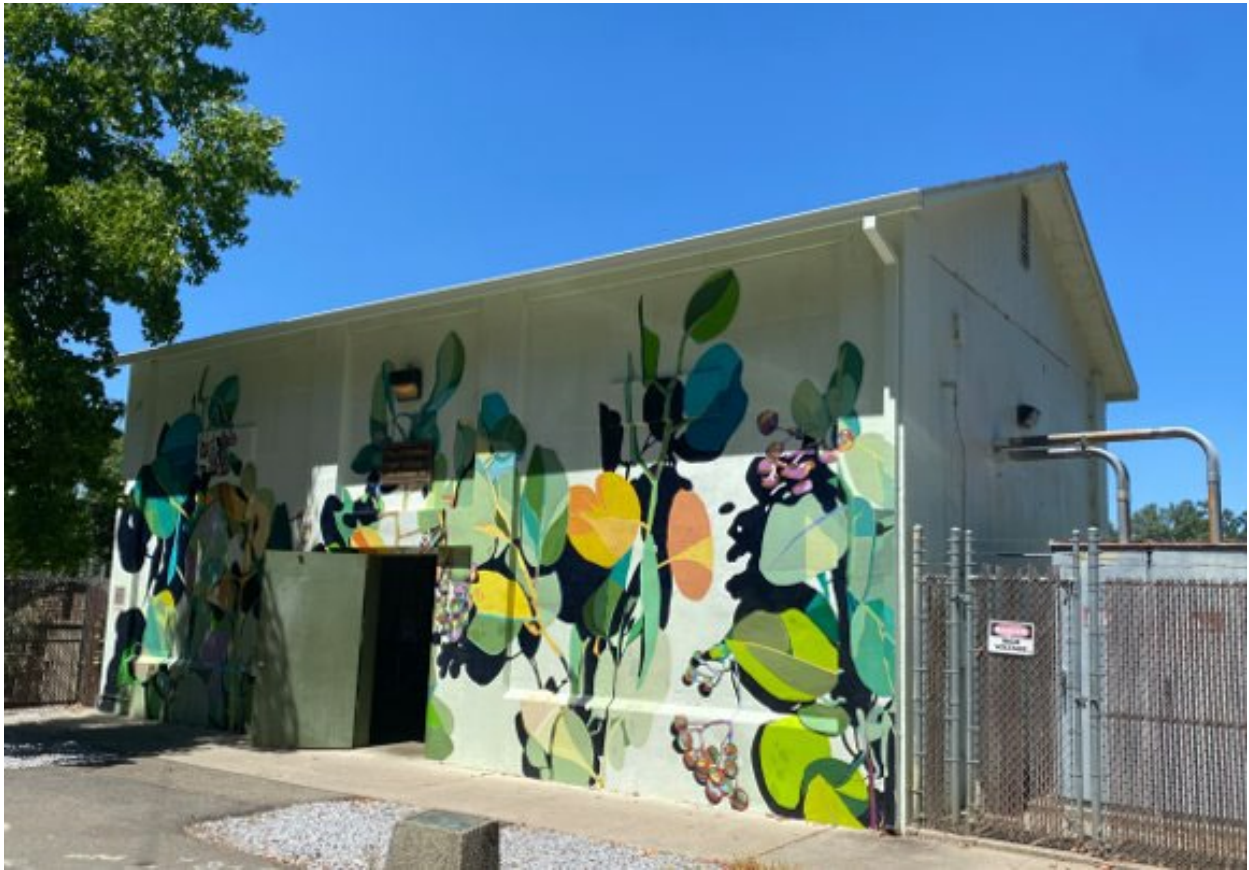
Figure 2. Landside Photograph of Existing PS1
