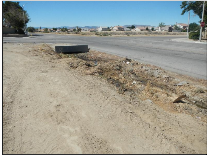
8. Additional view of storm water drainage along 25 th Street East
