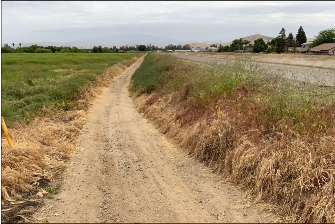
Figure 4-7 Access road alongside canal levee, facing northeast.
