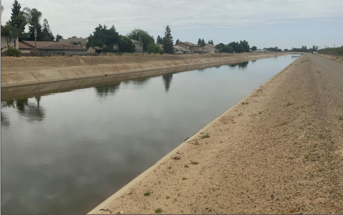
Figure 4-12 Overview of Friant-Kern Canal from northeast corner of APE, facing southwest.
