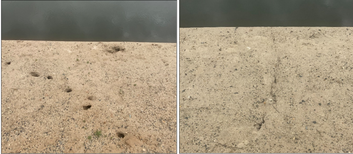
Figure 4-11 Representative examples of north bank conditions, with animal burrowing at left and erosion at right, facing southeast.
