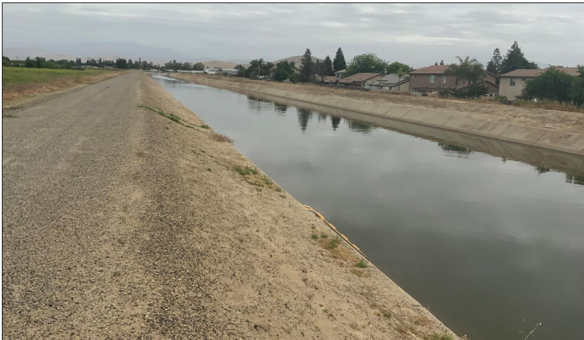
Figure 4-8 Overview of Friant-Kern Canal from southwest corner of APE, facing northeast.
