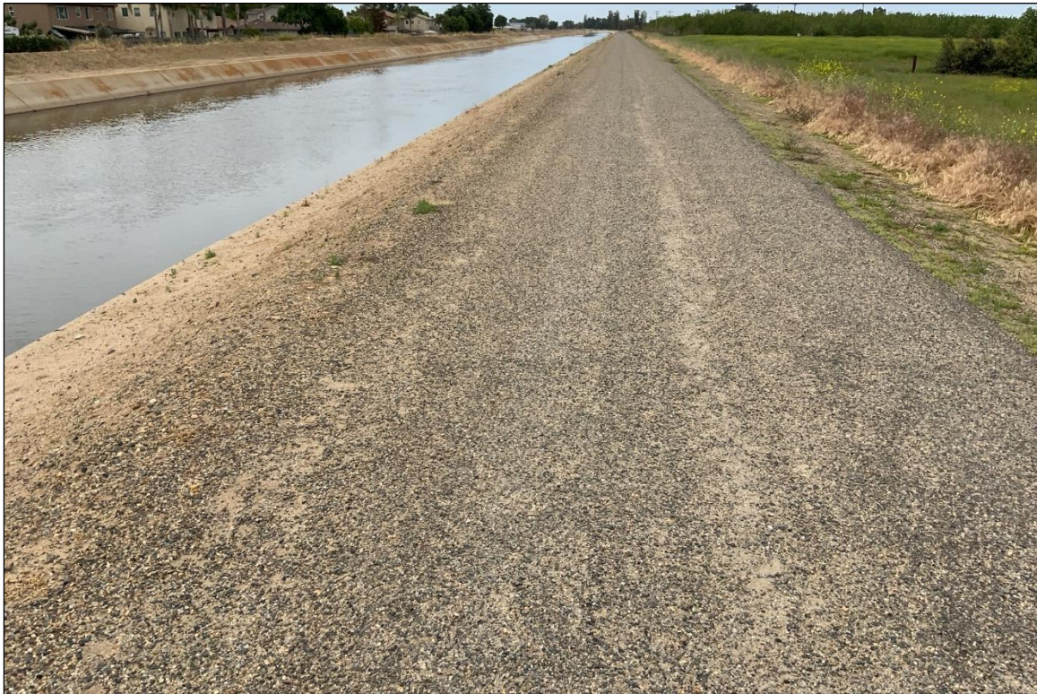
Figure 4-6 Surveyed canal levee road from northeastern portion of APE, facing southwest.
