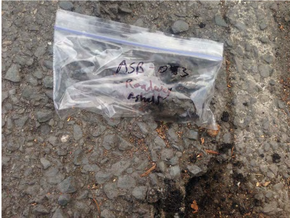
Photo 7. Sample ASB-03 taken from asphalt roadway along the east side of the center median
