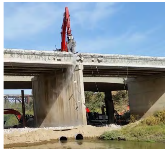
Figure 2: Example of Stream diversion and Earthen Work Pad for Bridge Removal
