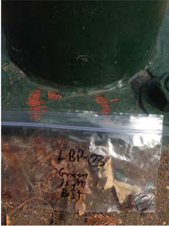
Photo 5. (left) Sample LBP-03 taken from the green paint on the light post in the center median; (right) photo showing light post in the center median
