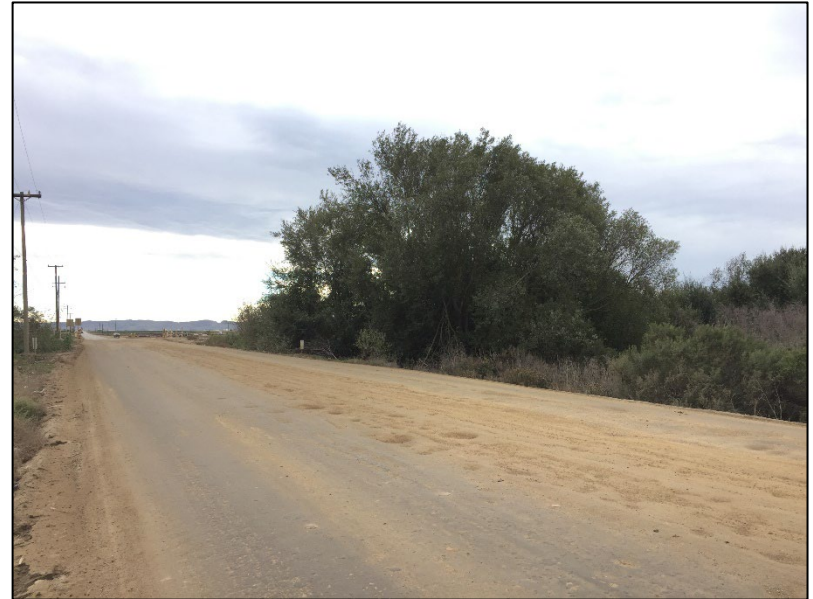
d. Embankment fill crossing near the southern levee, facing north
