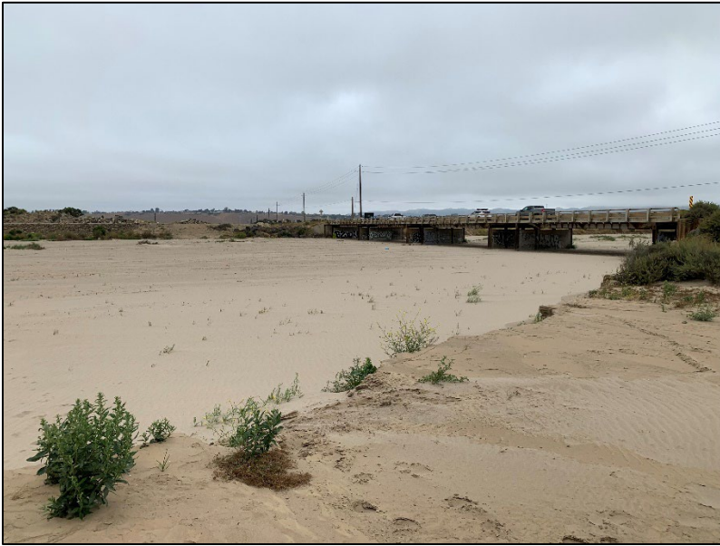
a. Existing bridge (right) and embankment fill (left background)
