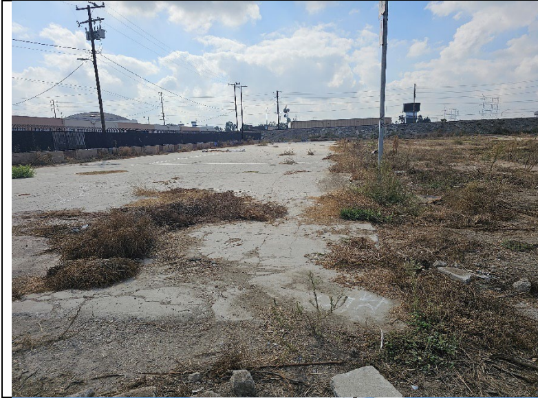
Photo 33: From northwest corner of structure pad, facing south, across pad.
