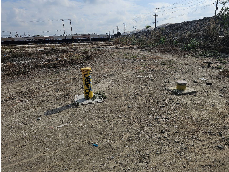
Photo 14: From southwest quadrant of property, facing east, toward groundwater monitoring wells.
