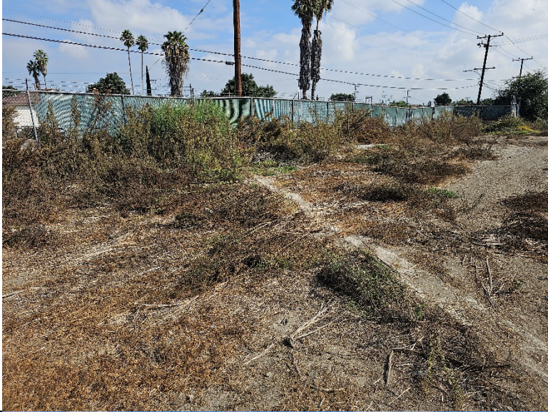
Photo 21: From north-central area of site, facing northeast, toward Shull Street. Cinder block footings of former wall or fence. Wall may have served as property boundary for a former residence or other structure, per the 1954 historic aerial survey image, but was later used as a storage yard.
