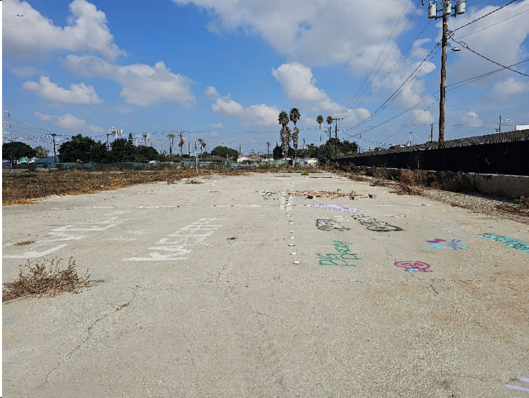
Photo 38: From south end of structure pad, facing north.
