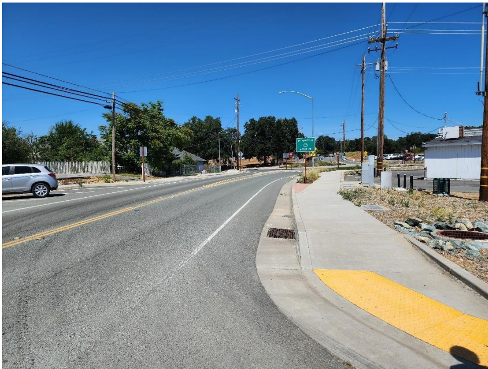
Looking East onto Main Street
