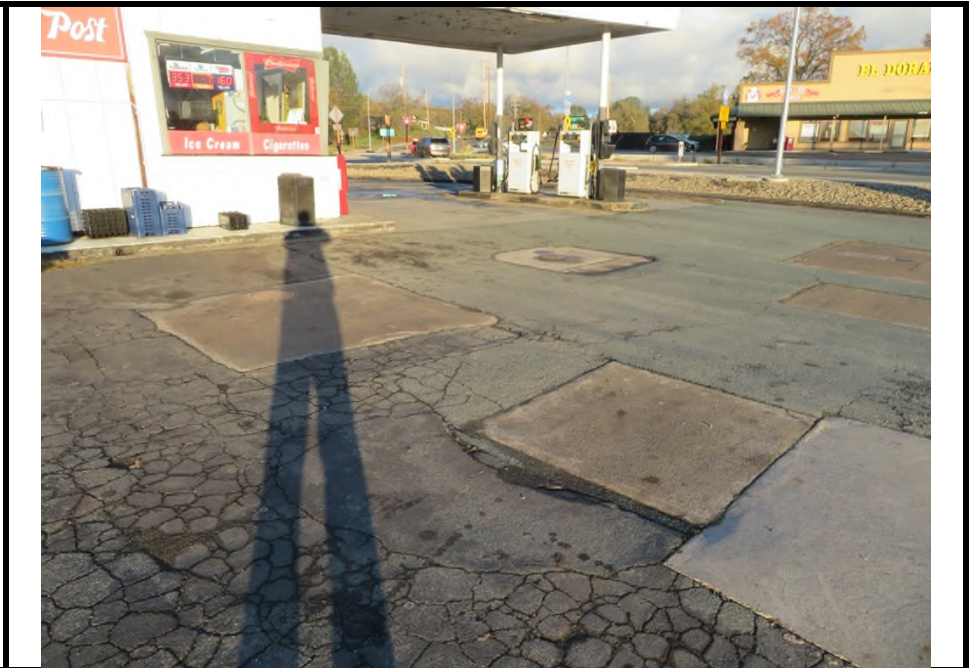
ESA Photo 7: View of the UST locations at 18725 Highway 49.
