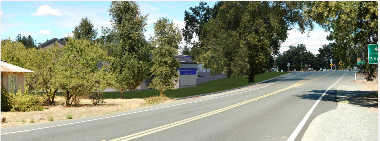
Figure 4.1-6b. Viewpoint 1 After Project
