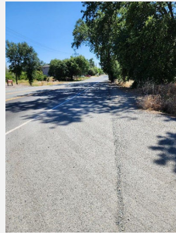
Figure 4.17-1f. SR-49 / Project Access 3 (South). Looking South onto SR-49
