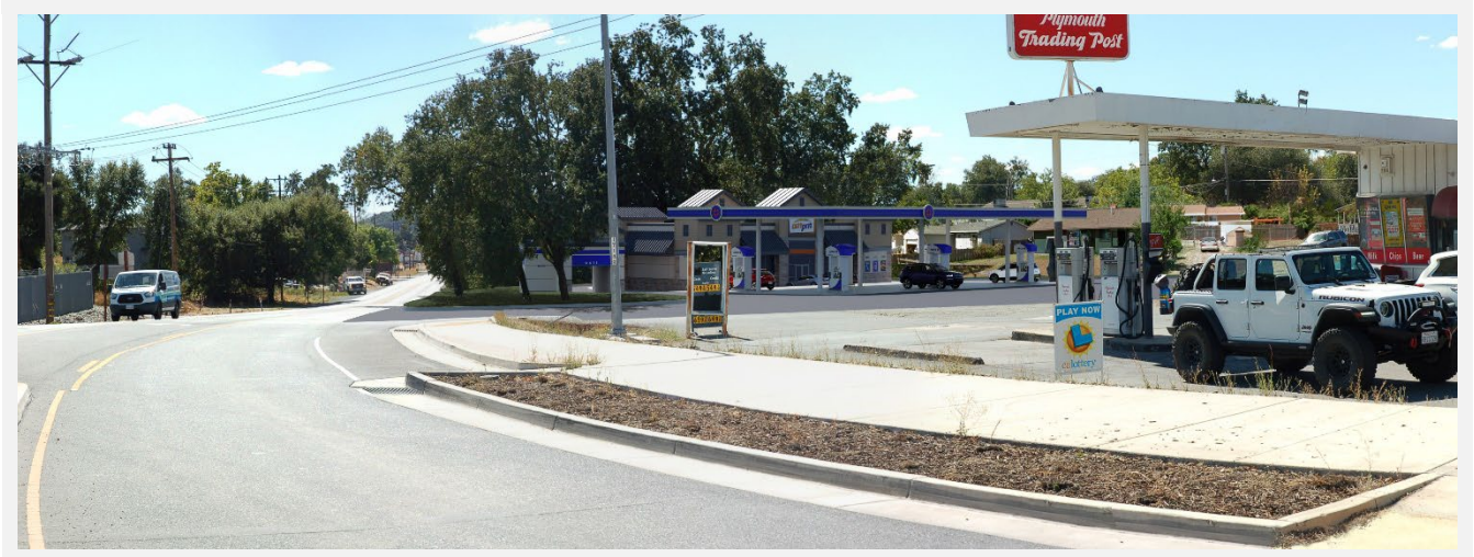
Figure 4.1-6d. Viewpoint 2 After Project
