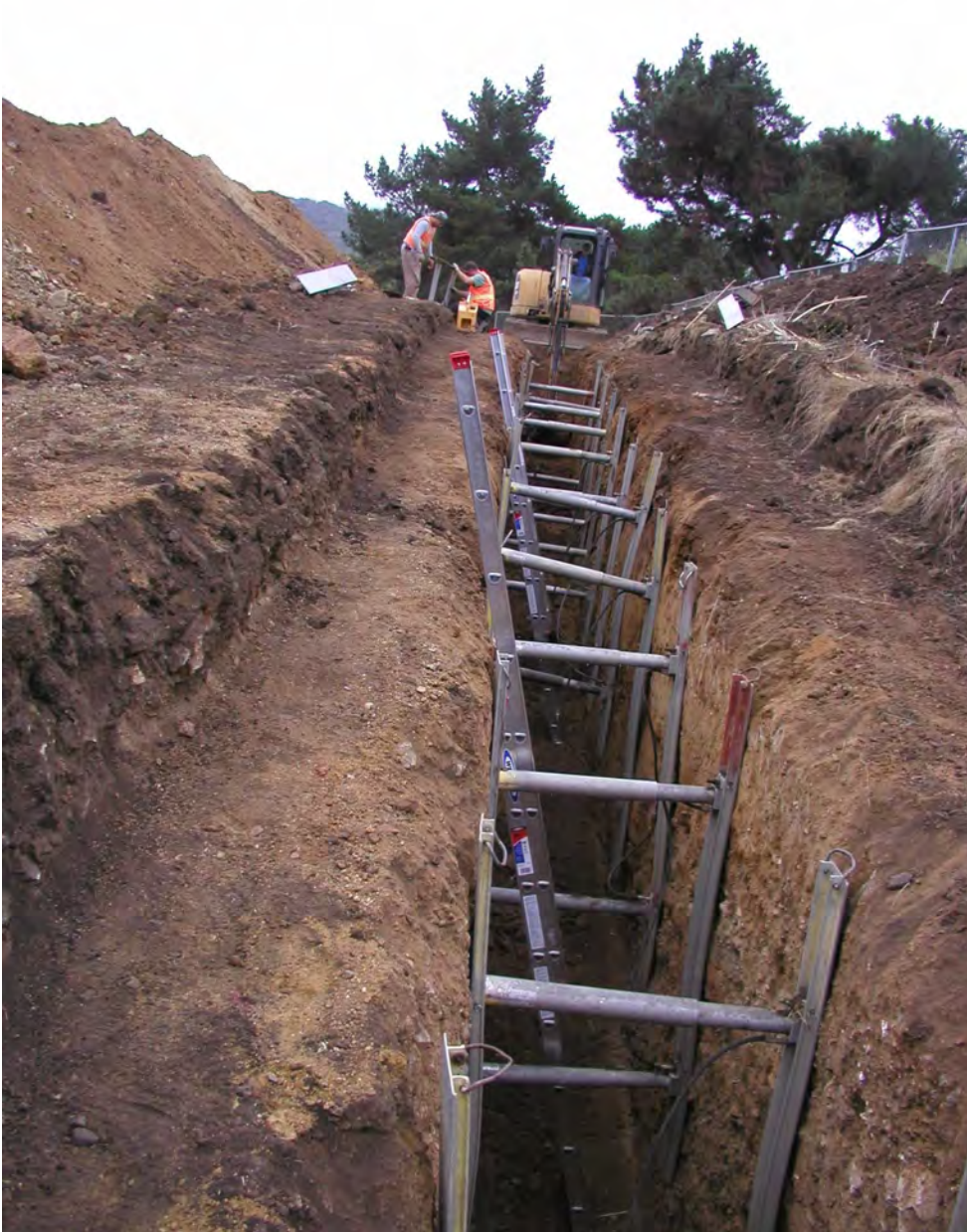
Photograph No. 8: Trench A during excavation. View to southwest.
