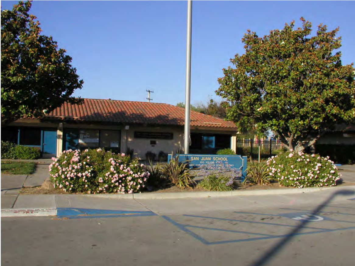
Photograph No. 1: View to east. Office building (Building A).
