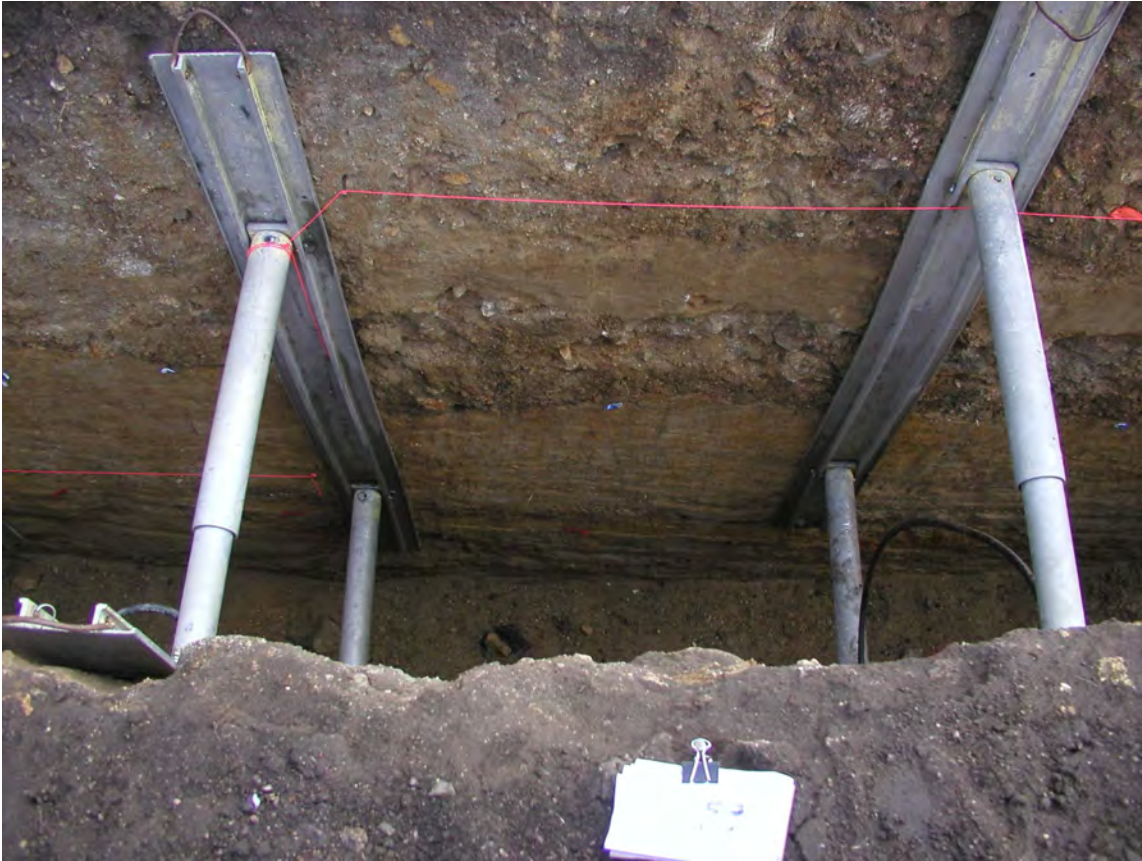
Photograph No. 11: Trench A, station 45.
