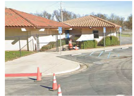
④ Facing northeast at the southeastern end of the project site.
