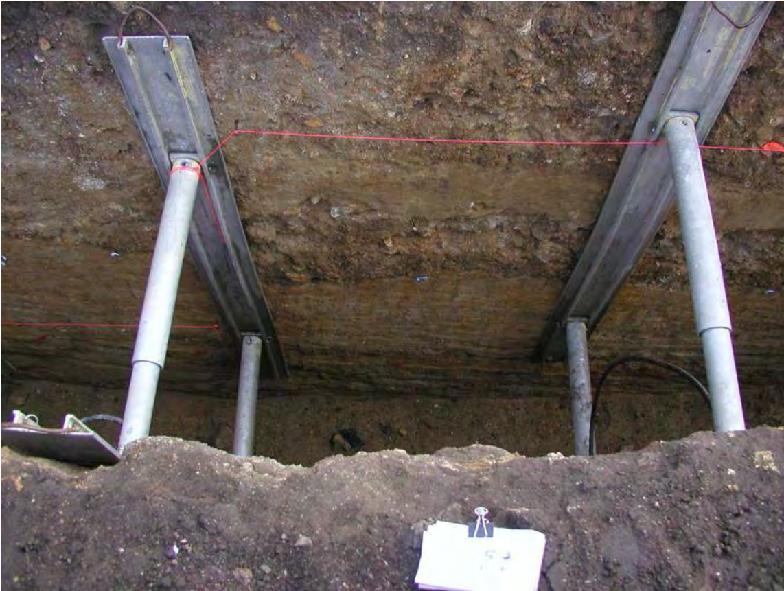
Photograph No. 11: Trench A, station 45.
