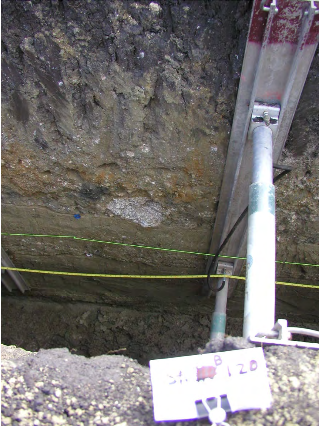
Photograph No. 15: Trench B. Station 120.
