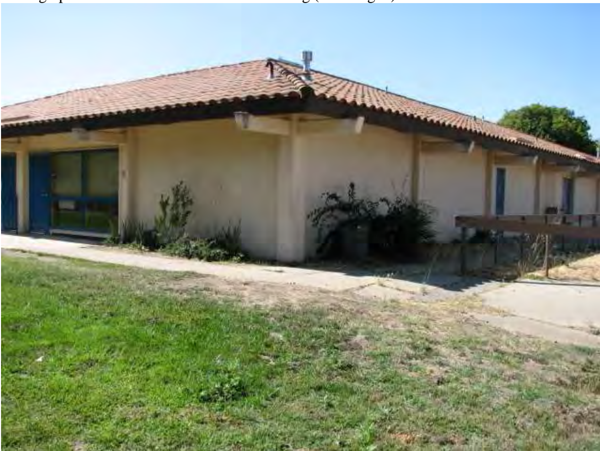
Photograph No. 2: View to south. Classroom building (northeast corner Building D).
