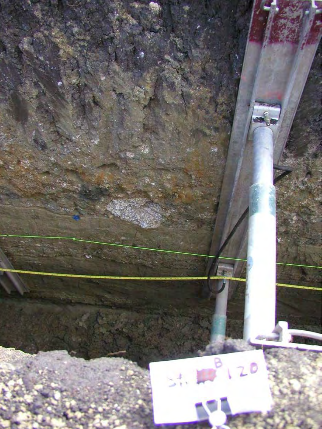
Photograph No. 15: Trench B. Station 120.
