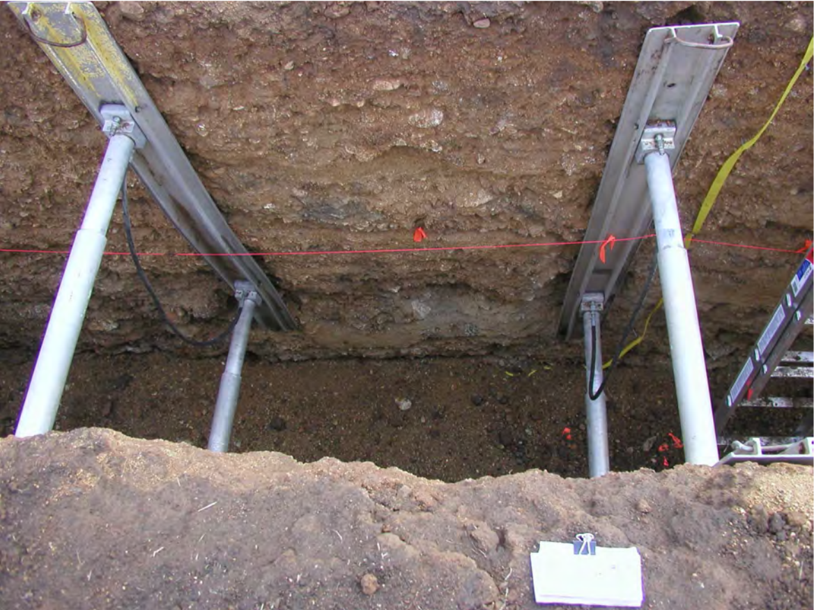
Photograph No. 9: Trench A, station 133.
