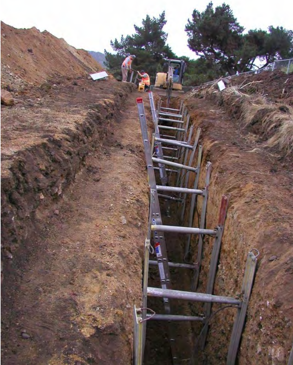
Photograph No. 8: Trench A during excavation. View to southwest.
