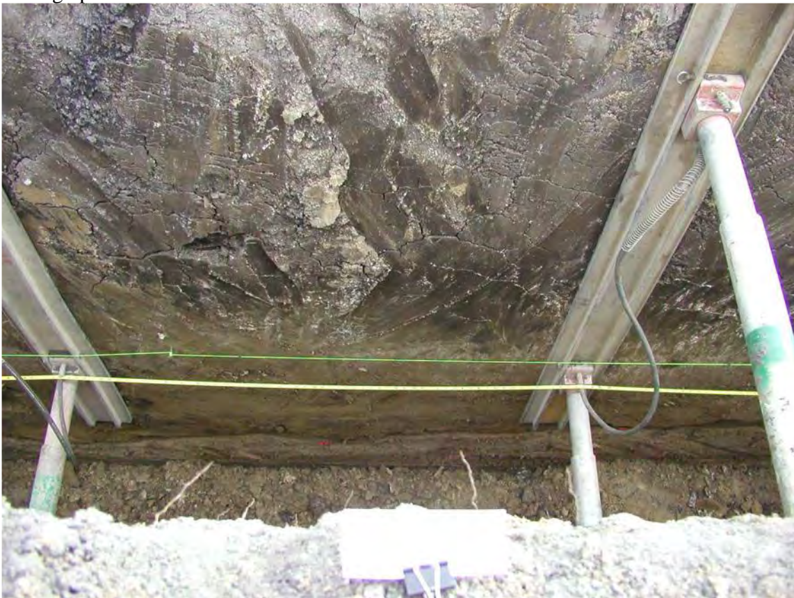
Photograph No. 17: Trench B. Station 250.
