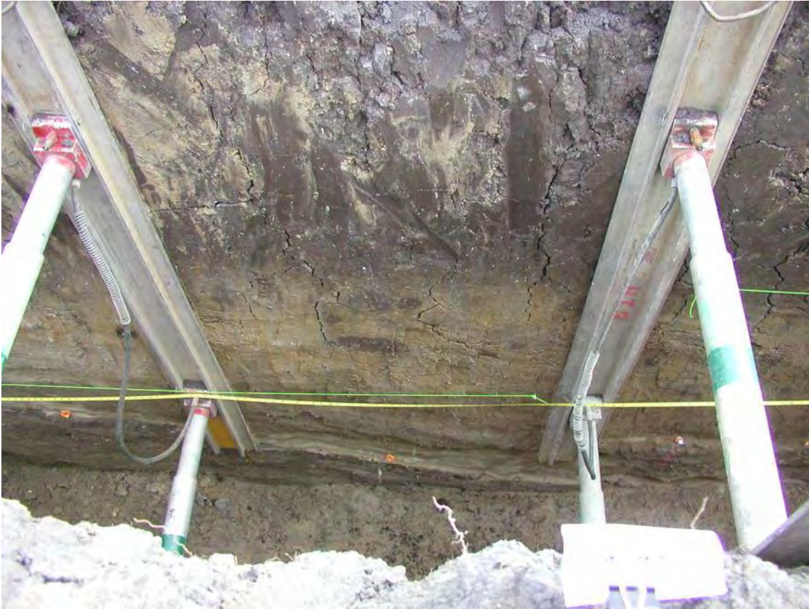
Photograph No. 16: Trench B. Station 150.
