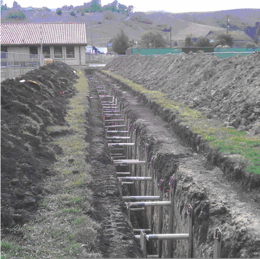
Photograph No. 14: Trench B, View to southwest.
