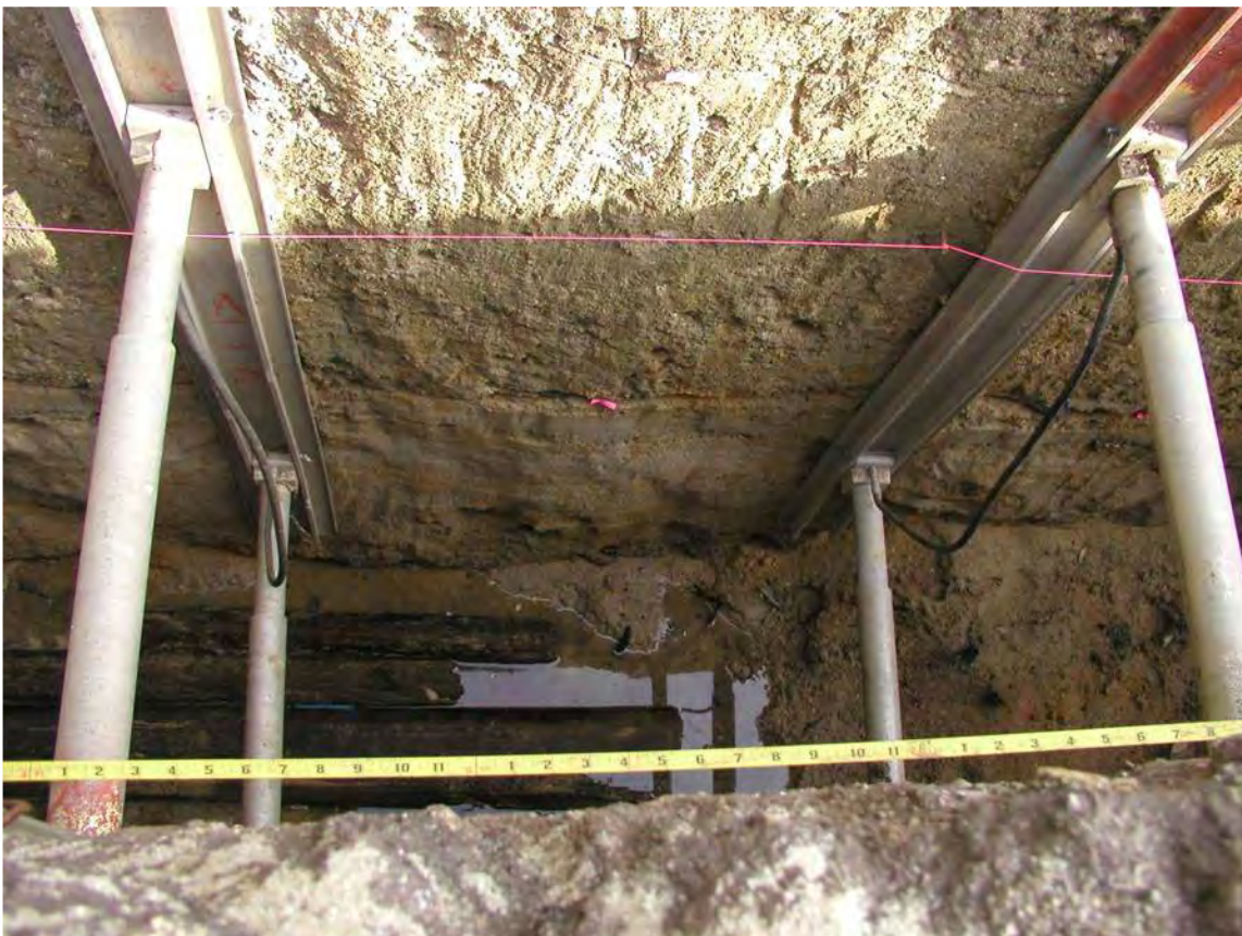
Photograph No. 12: Trench A, station 6.
