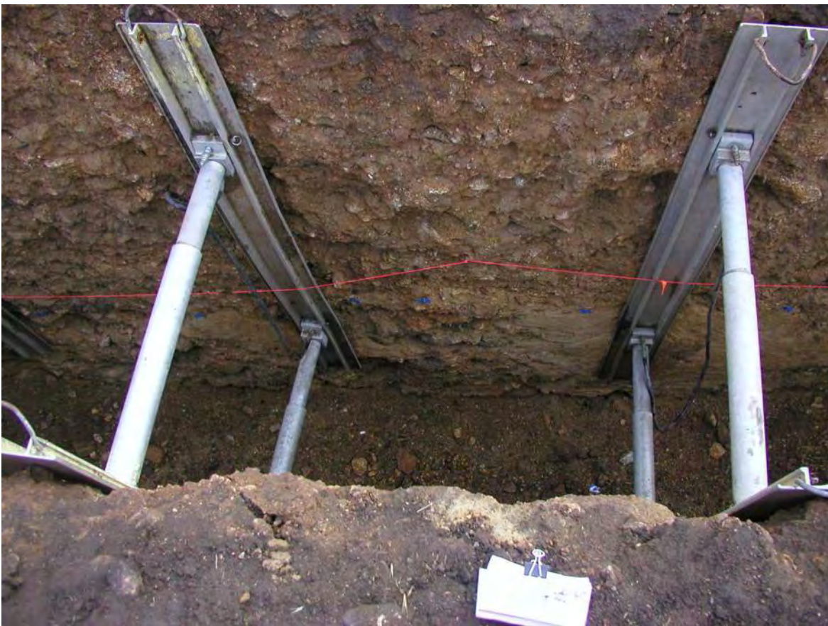
Photograph No. 10: Trench A, station 115.
