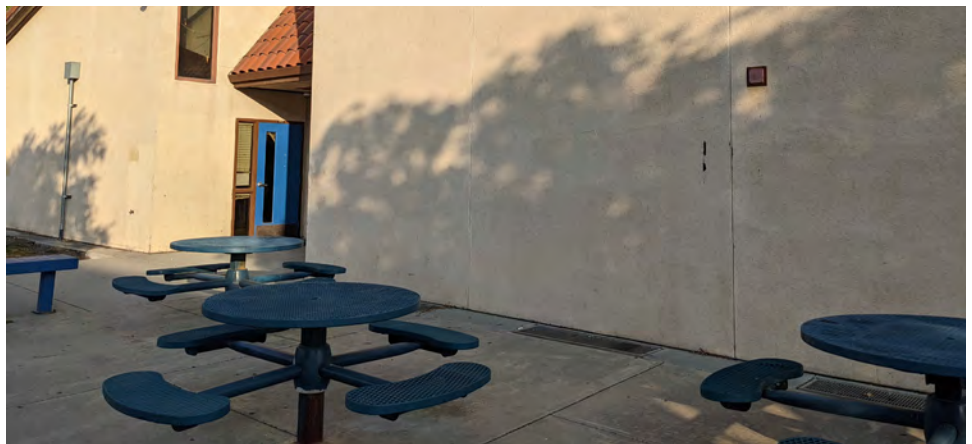
Existing Classroom Buildings & Courtyard
