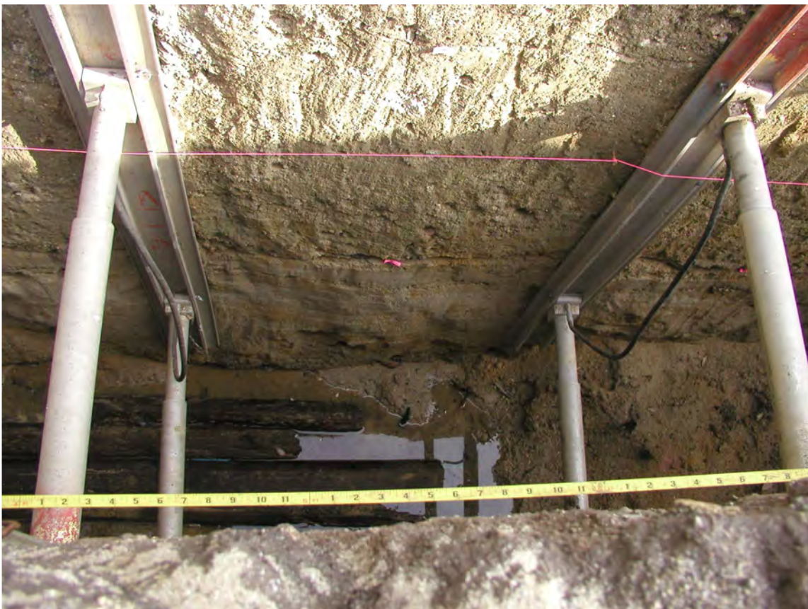
Photograph No. 12: Trench A, station 6.
