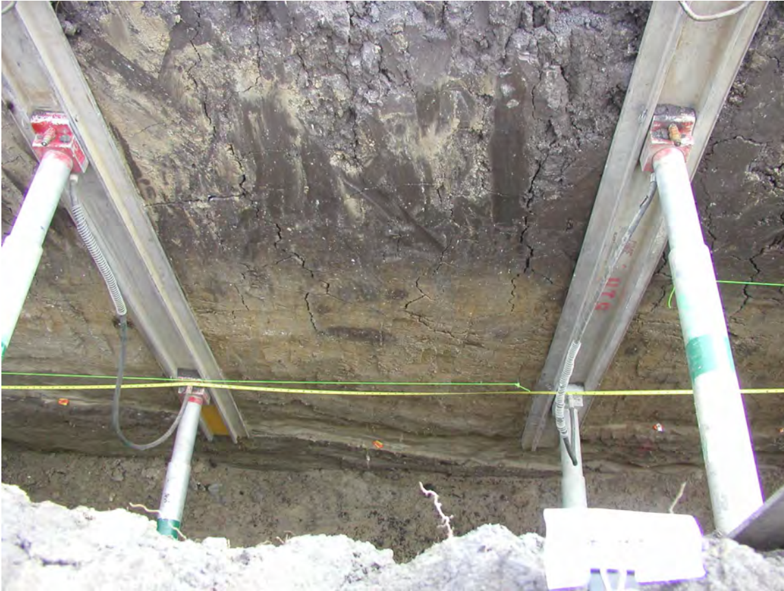
Photograph No. 16: Trench B. Station 150.
