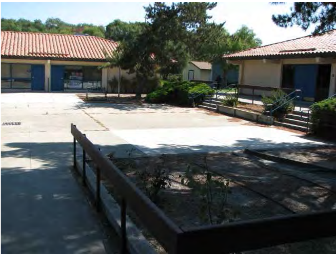
Photograph No. 4: View to east. Classroom building (Building E) on left and kitchen/multi-purpose building on right.
