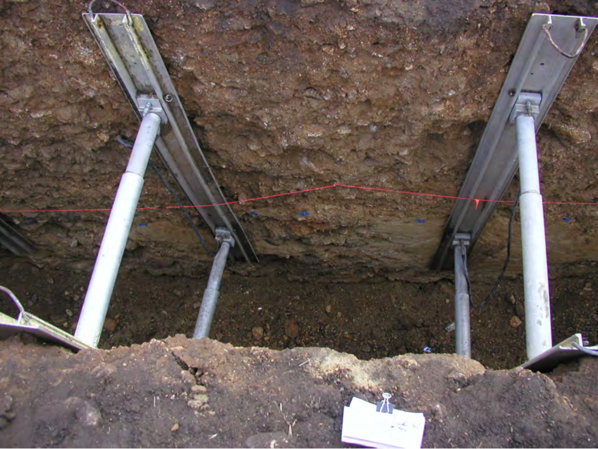
Photograph No. 10: Trench A, station 115.
