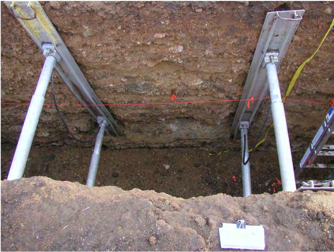
Photograph No. 9: Trench A, station 133.
