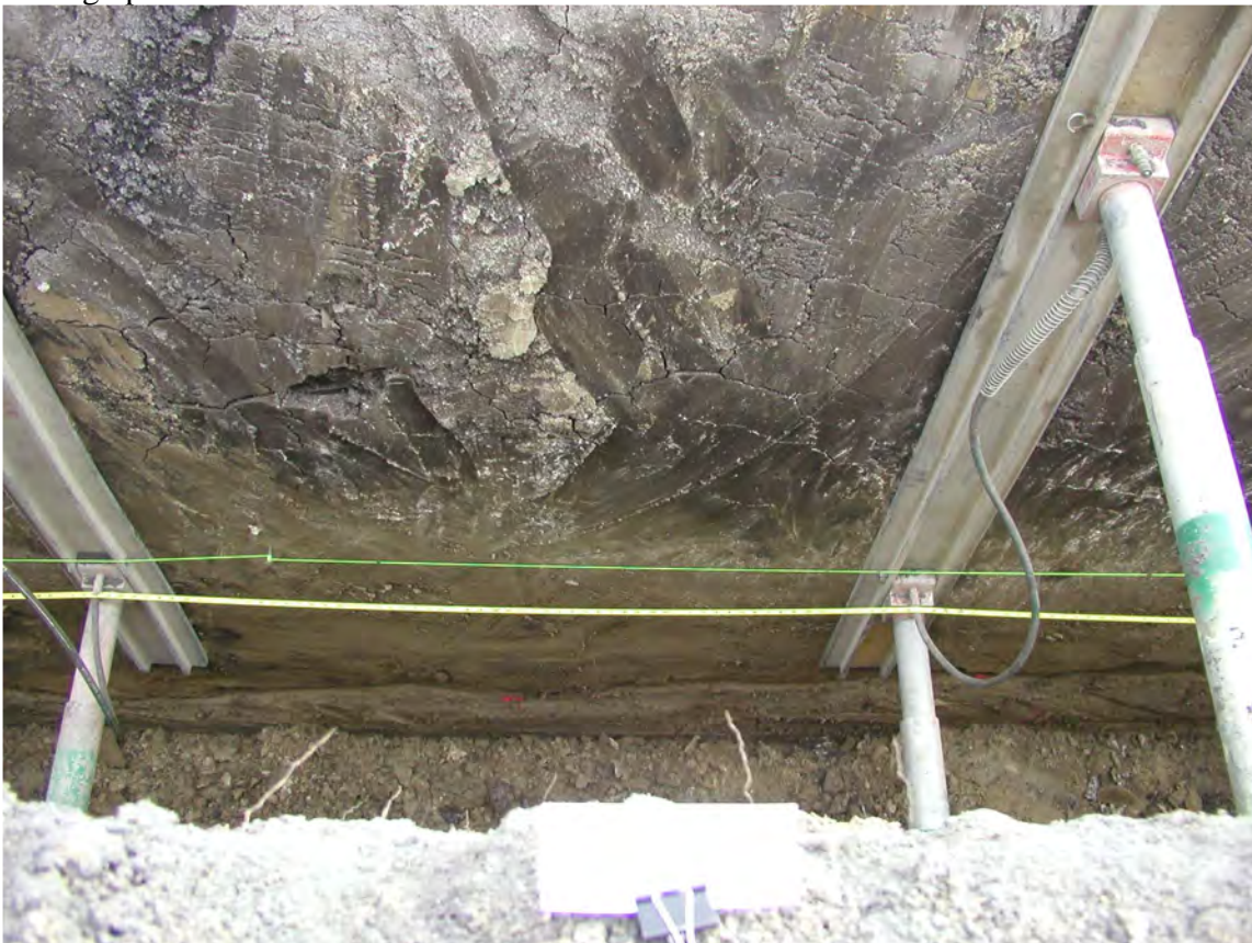
Photograph No. 17: Trench B. Station 250.
