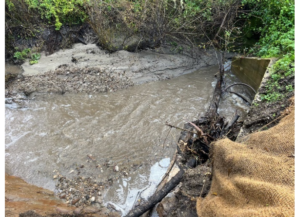
Photo 1. Lobitos Creek, facing southeast wingwall (1/23/2024).
