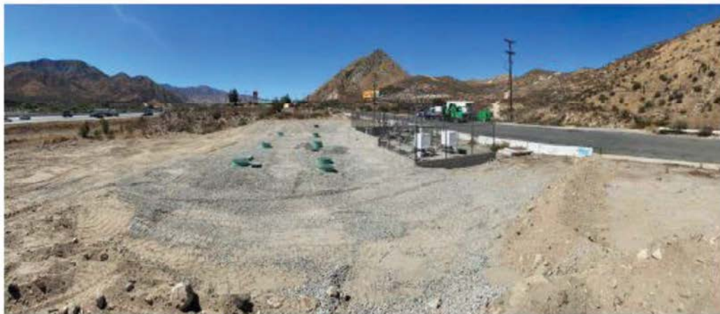
Photo 004: Off site Cajon Pass Wastewater Treatment Plant, facing northwest.
