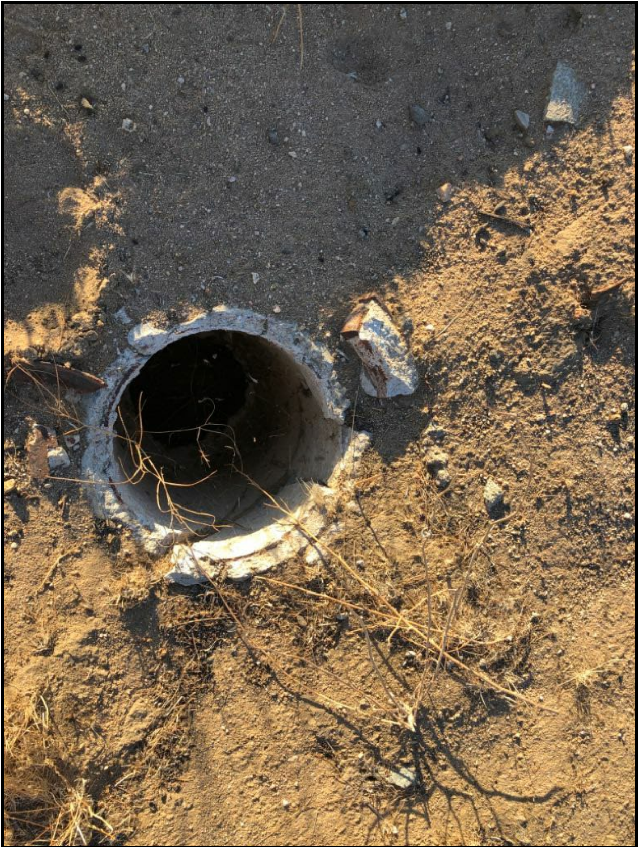
Figure 5. Open abandoned irrigation line. Photograph taken 9 October 2021.
