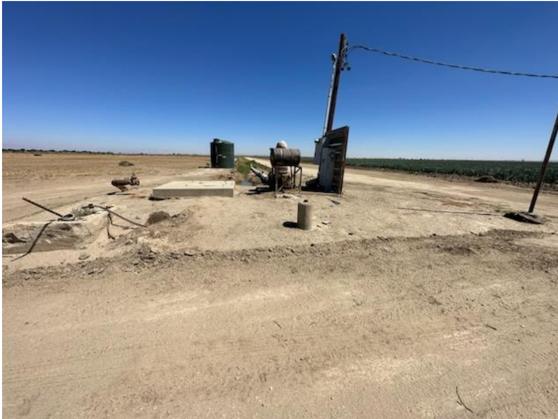
15. View of a groundwater well located near the middle of the Site.
