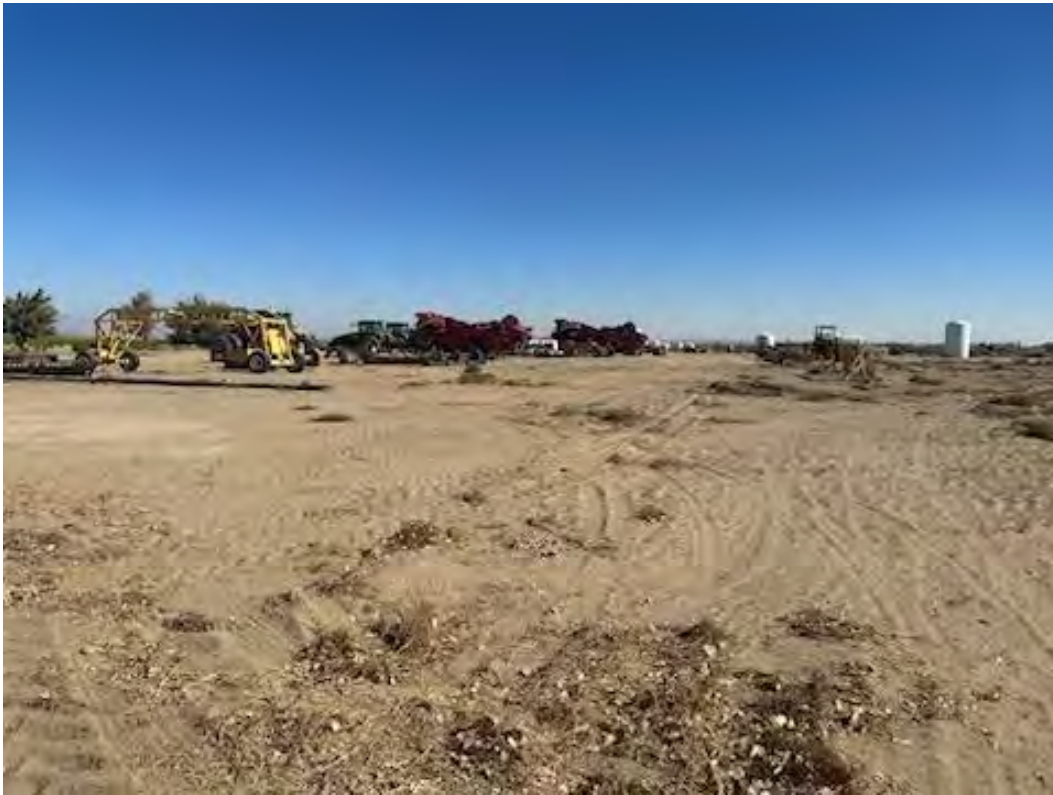
1. View looking at work area near the middle of the Site property.
