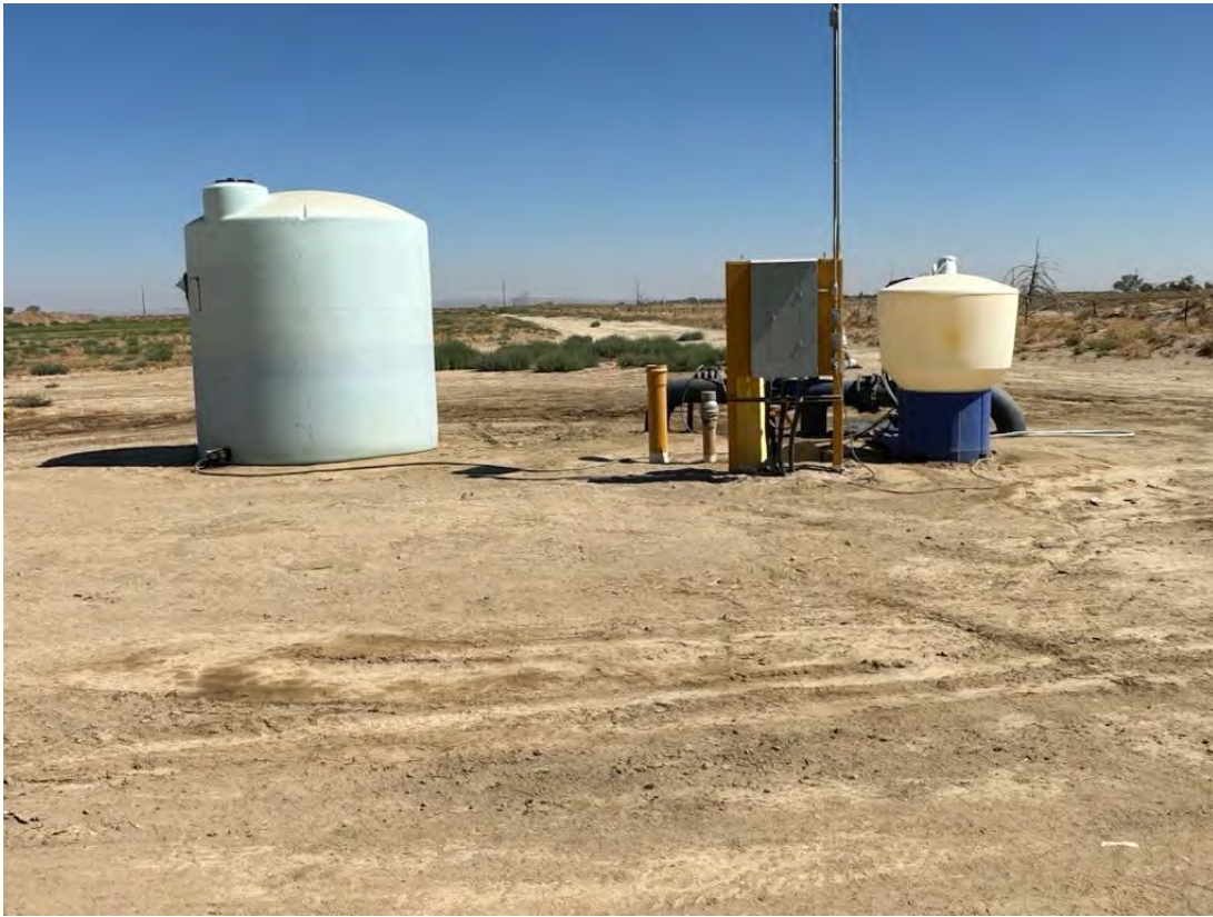
33. View of pumping station on the eastern portion of the Site.
