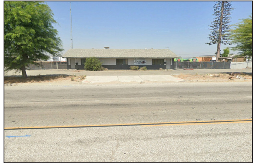
B. Looking at existing building at 2830 S Riverside Avenue from Riverside Avenue
