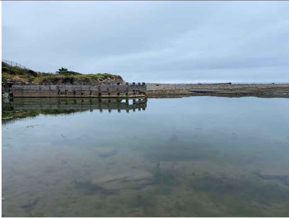
Photo 1. Creek conditions. Photo taken from northwest of bridge facing south. June 2023.
