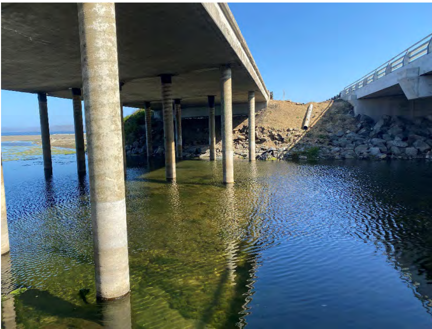
Photo 4. Toro Creek looking north under SB bridge toward RSP bank.
