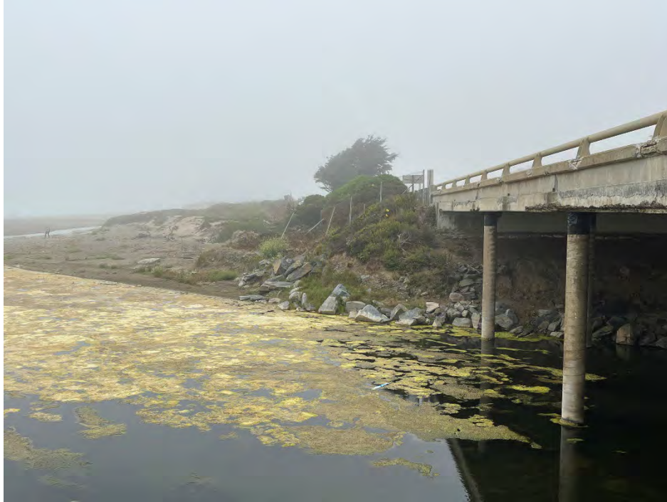
Photo 5. Creek conditions. Photo taken from southwest of bridge facing north. August 2023.
