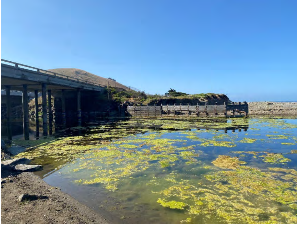
Photo 3. Creek conditions. Photo taken from northwest of bridge facing south. June 2023.
