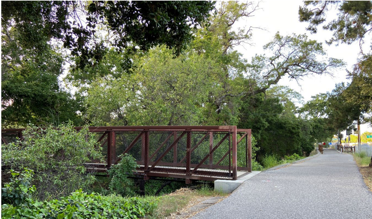
Photo 9. Pedestrian Bridge and paved trail.
