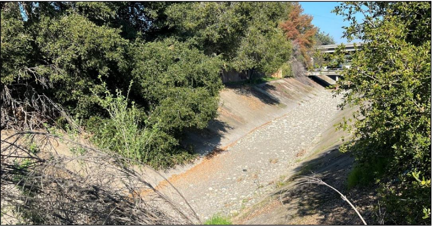
Photo 7. Viewing north along the existing Saratoga Creek channel towards Calvert Drive.
