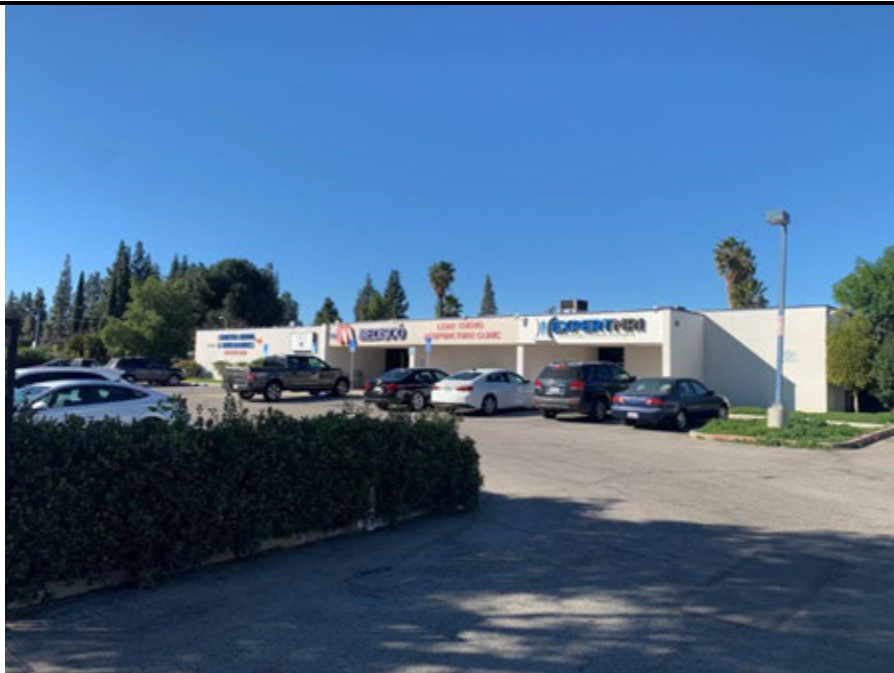
Photo 1: Exterior of building on Site looking southwest.
