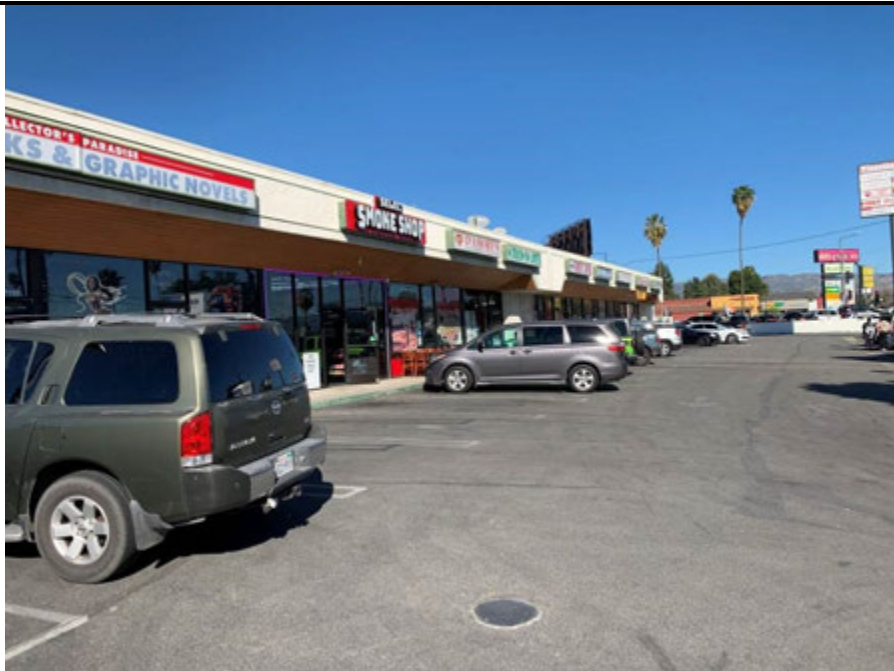
Photo 13: View of shopping center on north adjoining property, looking north (note the asphalt patch which marks the location of a former monitoring well in the parking lot).
