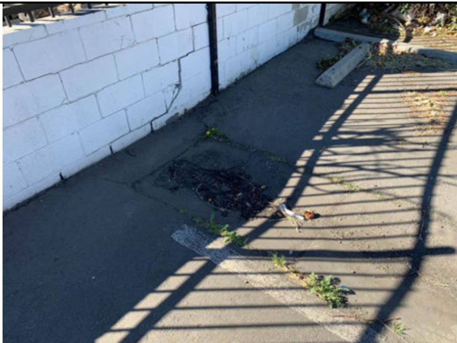
Photo 12: View of a catch basin in the parking lot, southwest of the building.
