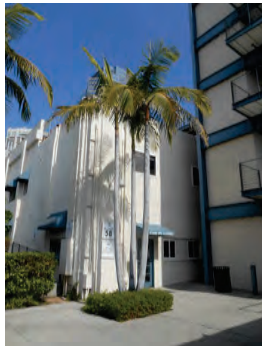
Tree 1380 – Archontophoenix cunninghamiana facing north
