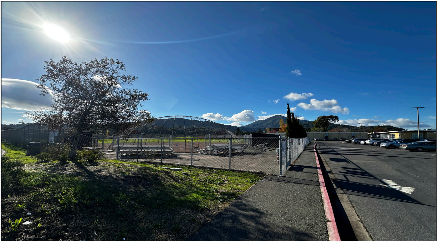
Intersection of Doherty Drive and Riviera Circle Looking South Towards Band Room and Athletic Fields
