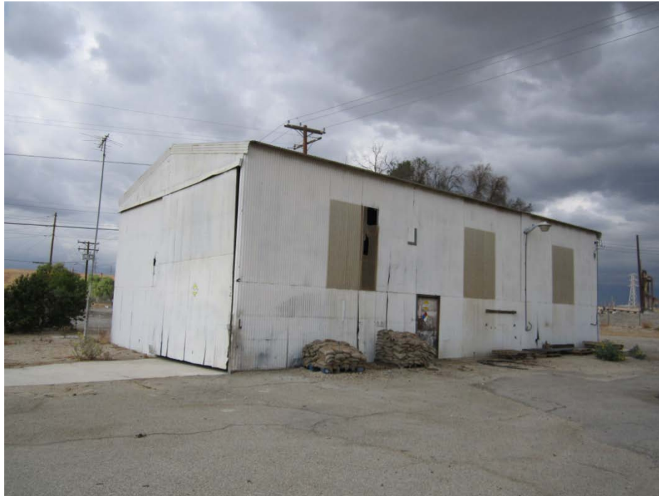
Feature 1 (AM-002): Southwest and Southeast Façade. Photo # 159
