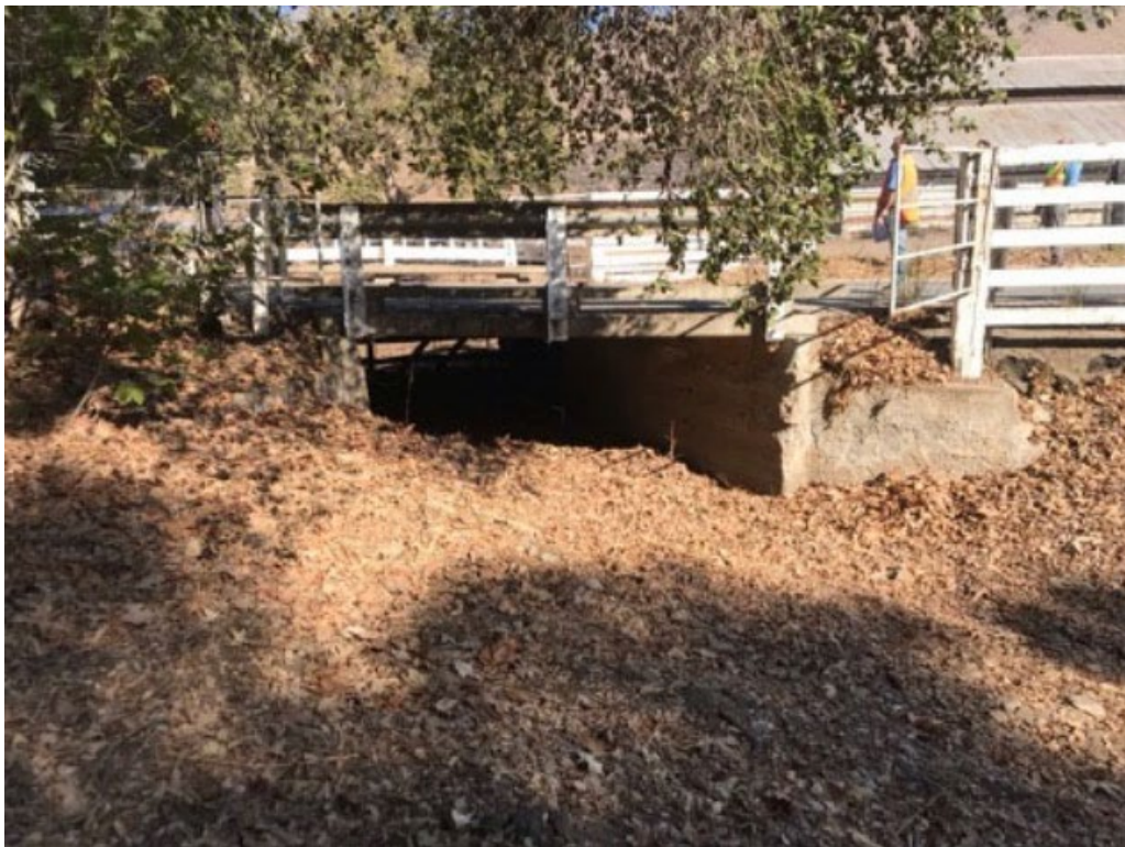
Figure 4: Bridge 304 Site Photo (Source: HDR | WRECO 2023)
