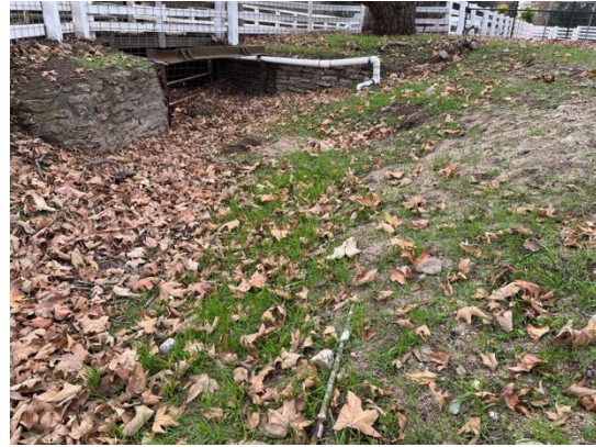
View of Bridge 305 including wingwalls and pipe. December 19, 2022. Facing south.
