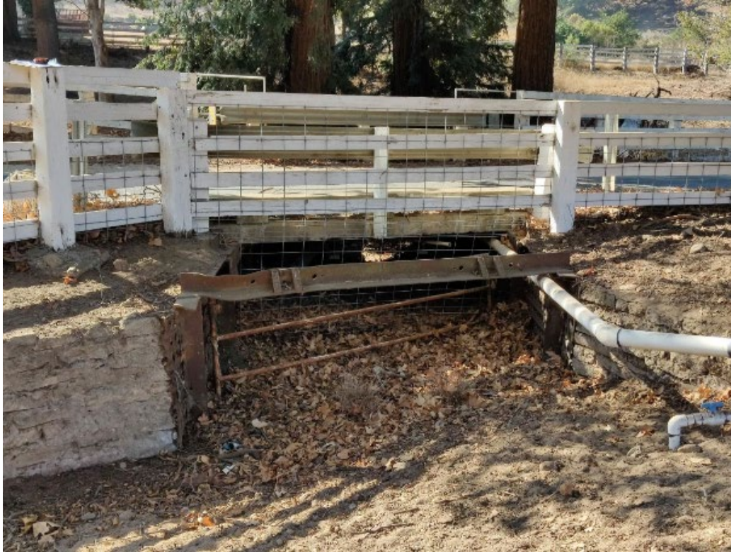
Figure 5: Bridge 305 Site Photo (Source: HDR | WRECO 2023)
