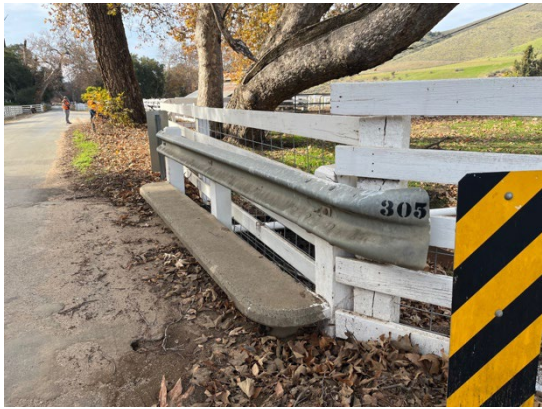
Guardrail on northern side of Bridge 305. December 19, 2022. Facing west-northwest.
