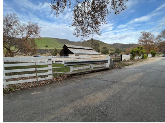
View of guardrail on northern side of Bridge 304 with barn in the distance. December 19, 2022. Facing northeast.
