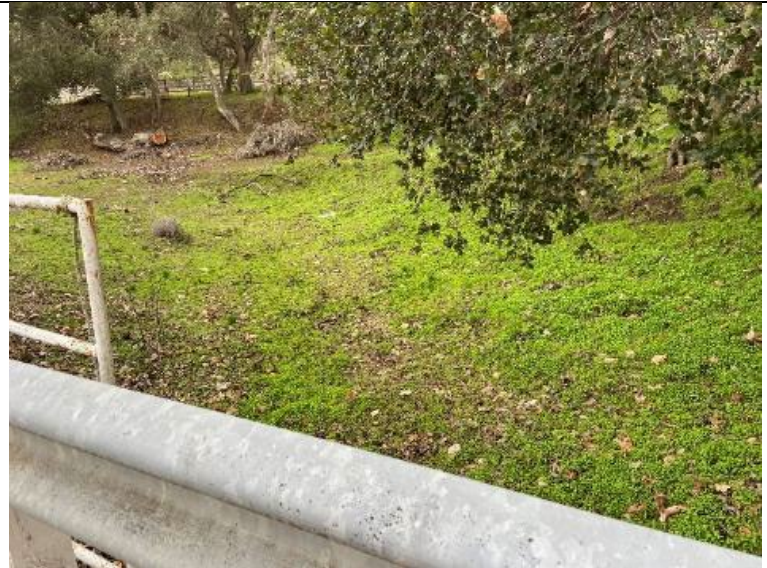
View from south side of Bridge 304, facing south-southeast.
