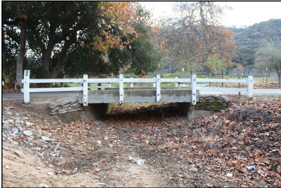
Photograph 2: Bridge 302; camera facing southwest; December 19, 2022.
