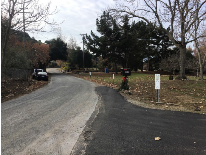
Bridge 302 Photo Point 1. Taken just outside of the northern boundary of Project site. Facing southwest.
