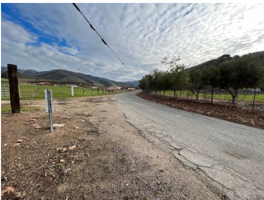
View of Chualar Canyon Road towards Bridges 303-305. December 20, 2022. Facing northeast.
