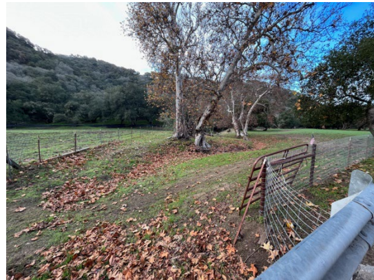
View of Chualar Creek drywash from Bridge 303. December 20, 2022. Facing south.
