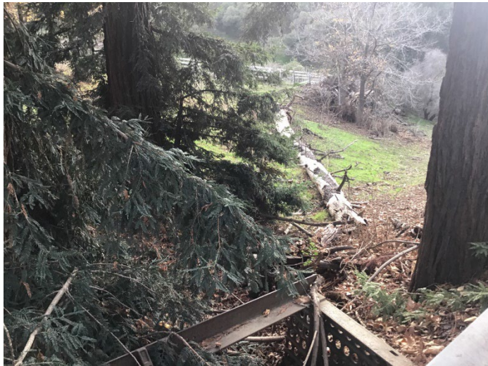
Bridge 304-305 Photo Point 3. View from south side of Bridge 305. Facing southwest, looking downstream in Chualar Creek.
