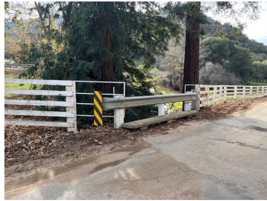
Guardrail on southern side of Bridge 305. December 19, 2022. Facing south-southwest.
