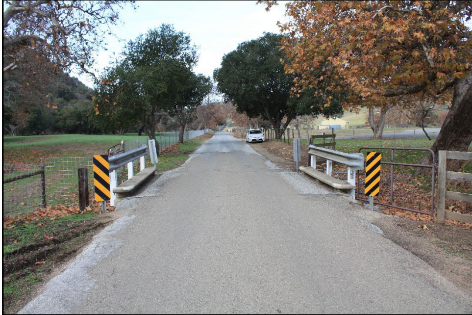
Photograph 6: Bridge 303; camera facing west; December 19, 2022.
