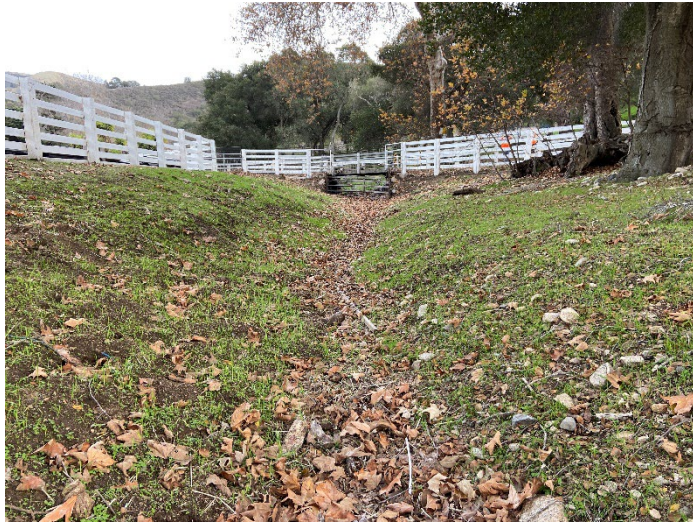
Bridge 304-305 Photo Point 5. Northern boundary of western region of Project site. Facing southeast, looking upstream within Chualar Creek.
