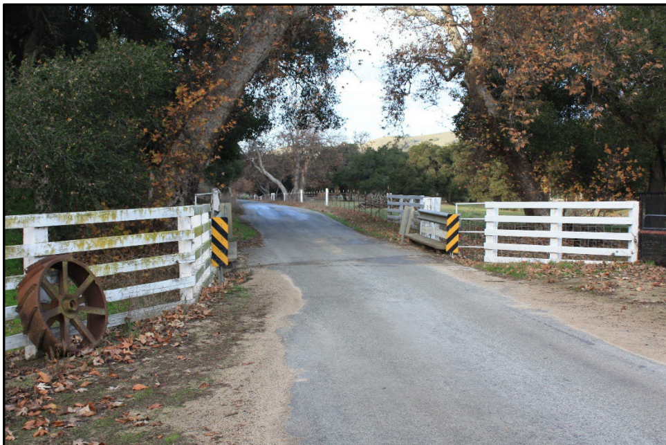
Photograph 9: Bridge 304; camera facing northwest; December 19, 2022.
