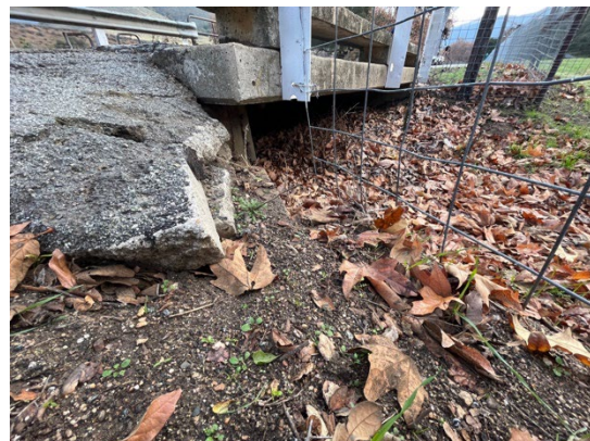
View of Bridge 303's structure from southwest corner. December 20, 2022. Facing northeast.
