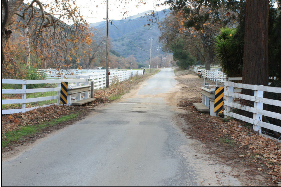
Photograph 12: Bridge 305; camera facing northeast; December 19, 2022.
