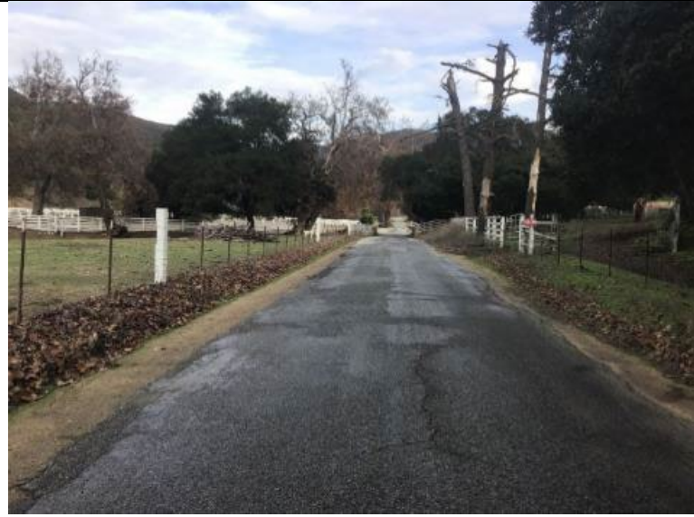
Western boundary of Bridge 304-305 Project site, facing east.
