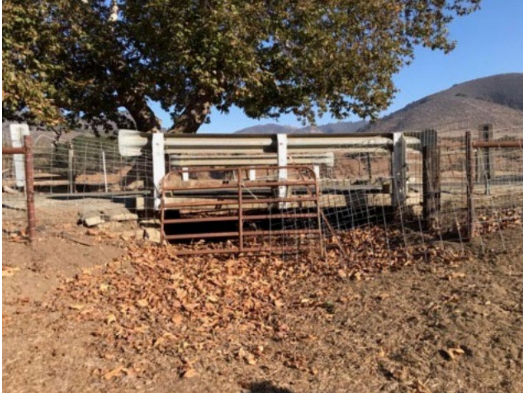
Figure 3: Bridge 303 Site Photo (Source: HDR | WRECO 2023)
