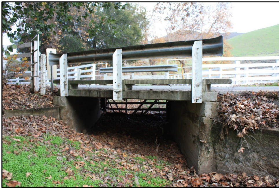
Photograph 11: Bridge 304; camera facing northwest; December 19, 2022.
