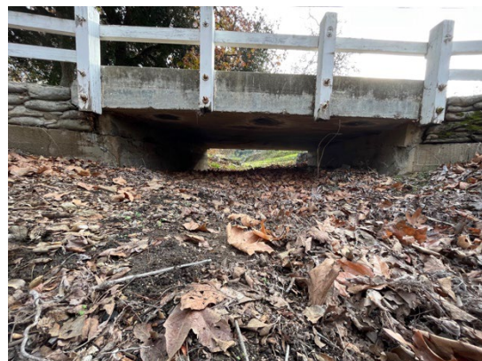
View under Bridge 302. December 20, 2022. Facing east.
