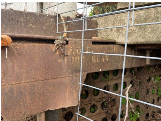
Closeup of lettering under Bridge 305. December 19, 2022. Facing northeast.
