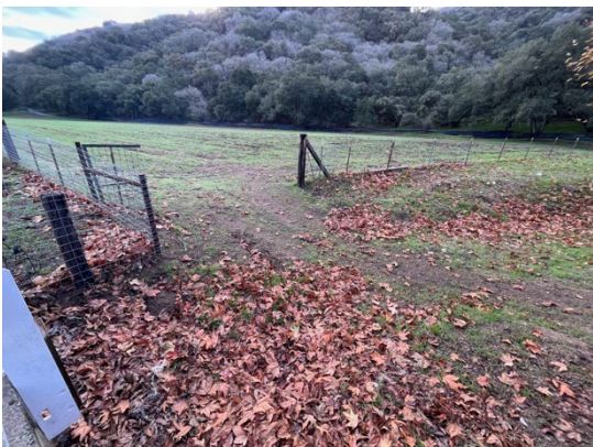
View of 4x4 access trail across Chualar Creek on southern side of Bridge 303. December 20, 2022. Facing southeast.
