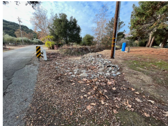
View of concrete and rock debris west of Bridge 302. December 20, 2022. Facing southwest.
