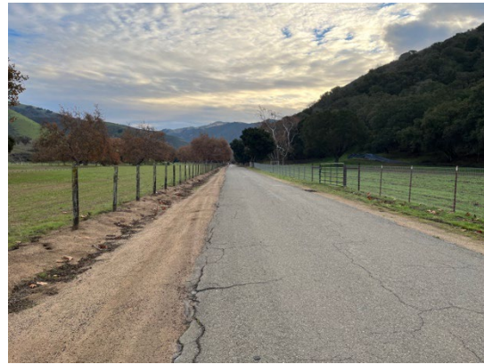
View of Chualar Canyon Road towards Bridge 304 from eastern APE boundary of Bridge 303. December 20, 2022. Facing east.
