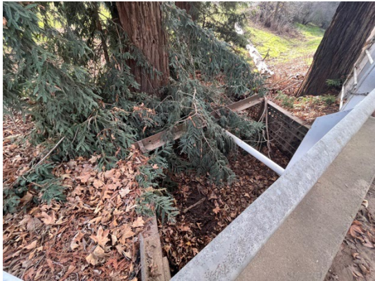
Overview of structure on southside of Bridge 305. December 19, 2022. Facing south-southwest.
