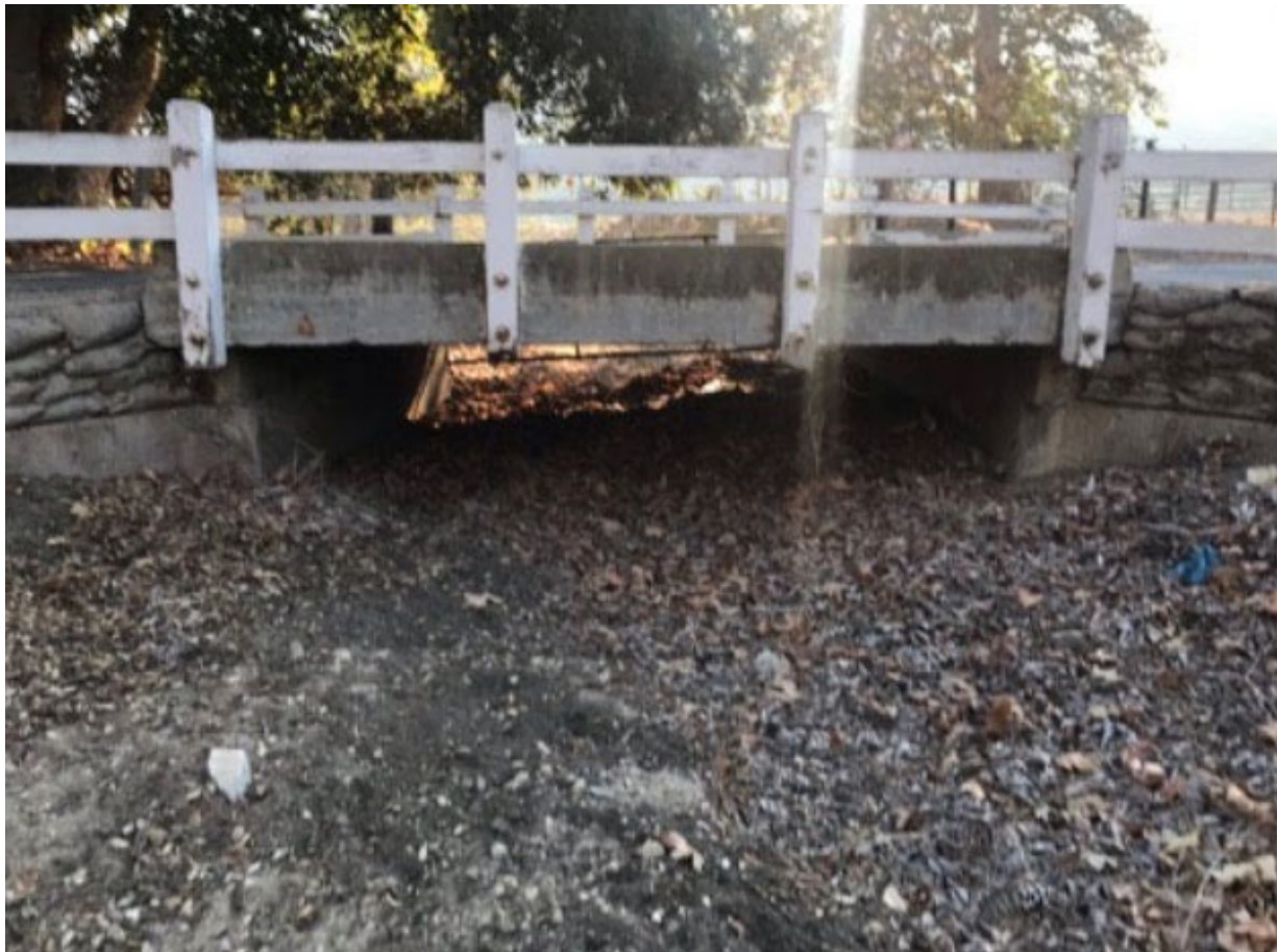
Figure 2: Bridge 302 Site Photo (Source: Source: HDR | WRECO 2023)
