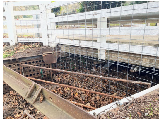
View of Bridge 305 from northwestern abutment wingwall. December 19, 2022. Facing northeast.
