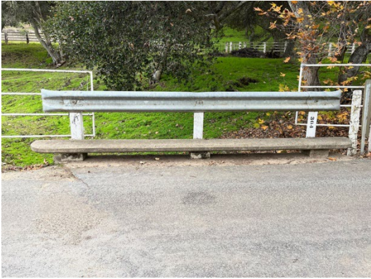
View of guardrail on southern side of Bridge 304. December 19, 2022. Facing south.
