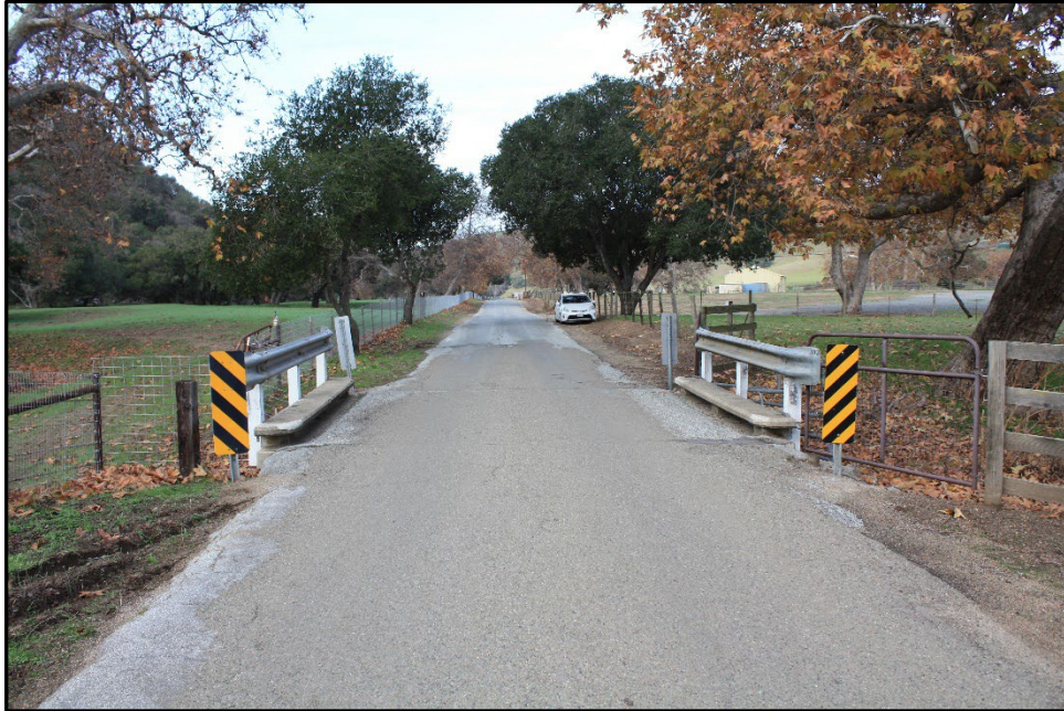
Photograph 6: Bridge 303; camera facing west; December 19, 2022.
