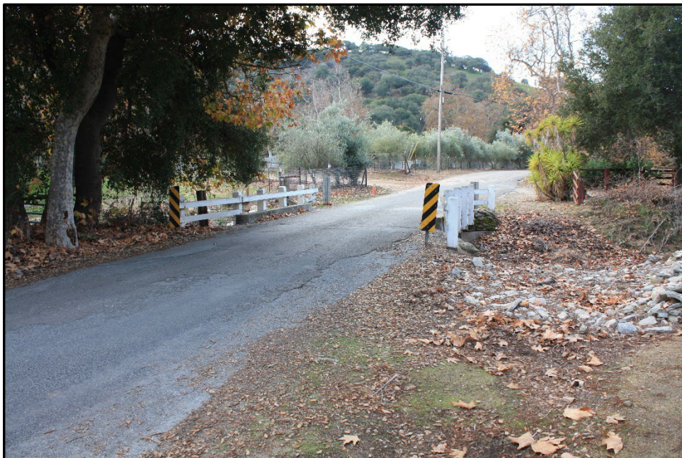
Photograph 5: Bridge 302; camera facing south; December 19, 2022.
