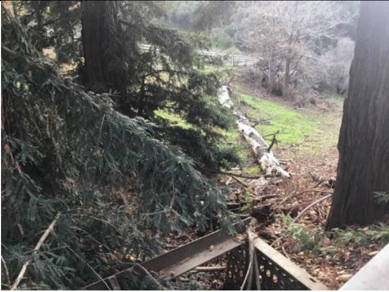
View from south side of Bridge 305, facing southwest.
