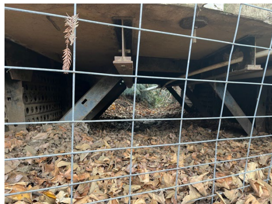
View under Bridge 305 through wire grate. December 19, 2022. Facing south.
