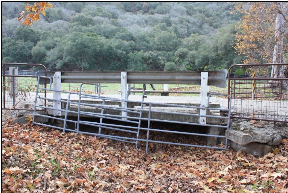
Photograph 7: Bridge 303; camera facing south; December 19, 2022.
