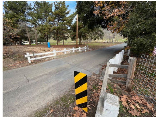
View of Bridge 302 over Chualar Creek. December 20, 2022. Facing northwest.
