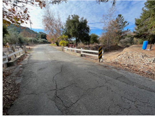
View of Bridge 302 from the north. December 20, 2022. Facing south.
