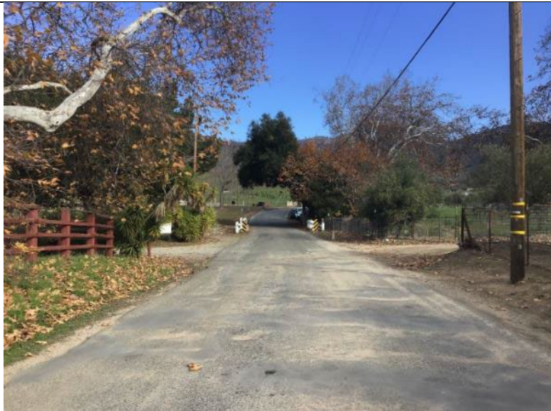
Southern boundary of Bridge 302 Project site, facing north-northeast.
