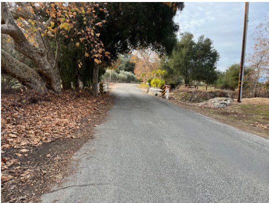
View of Bridge 302. December 20, 2022. Facing south.
