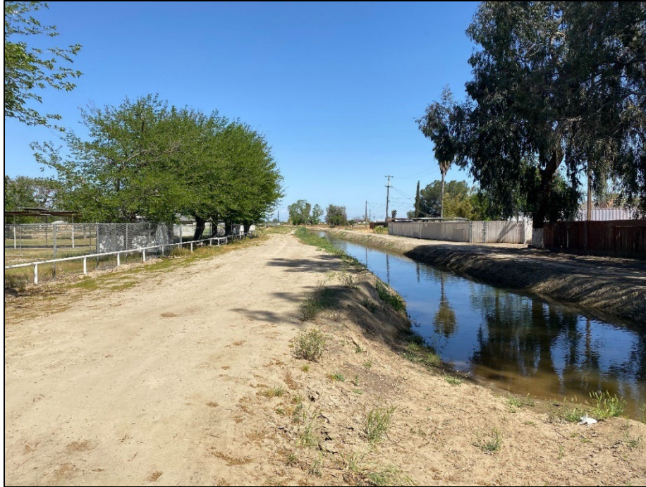
Figure 11. Overview of Project area showing Burrell Ditch, looking east.
