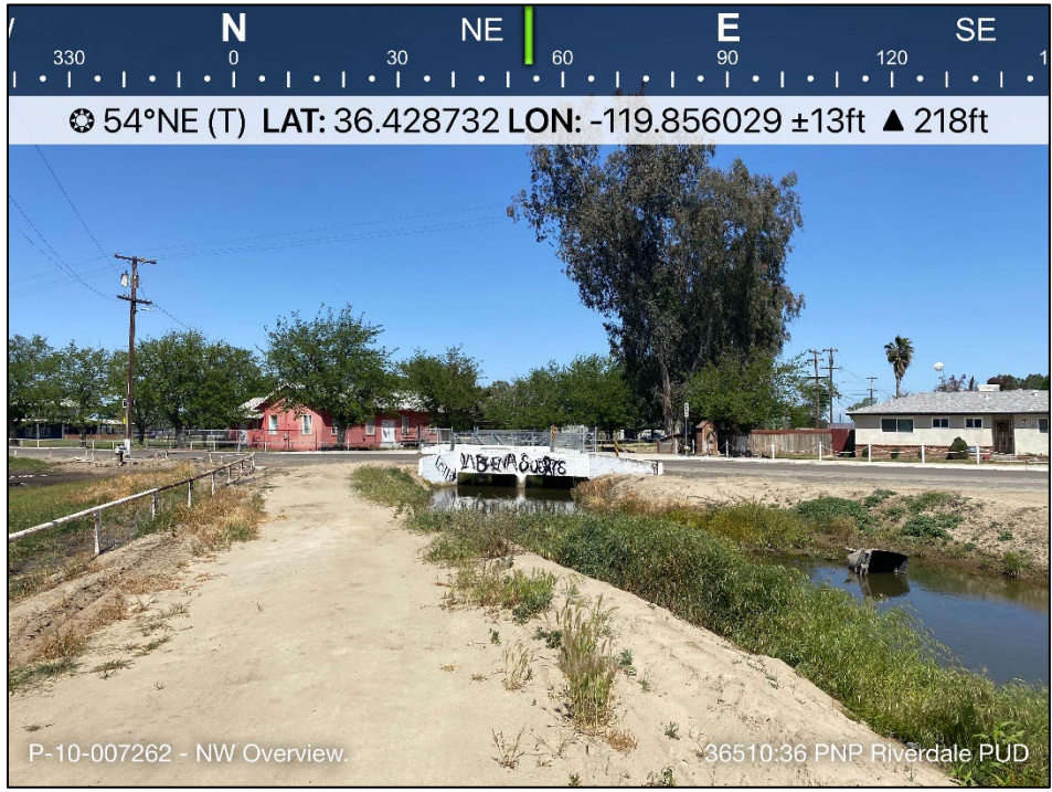
Figure 10. Overview of Project area showing existing infrastructure, looking northeast.
