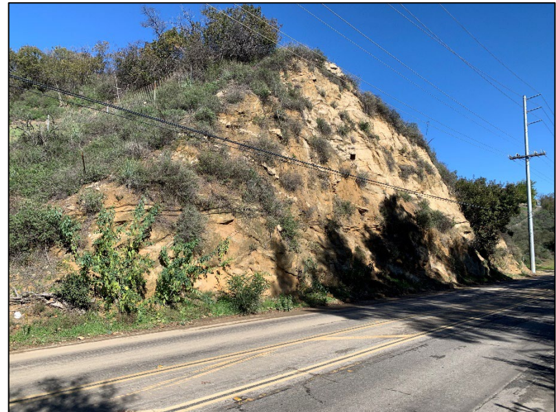
d. Slope to be stabilized with steel netting, near Viewpoint School
