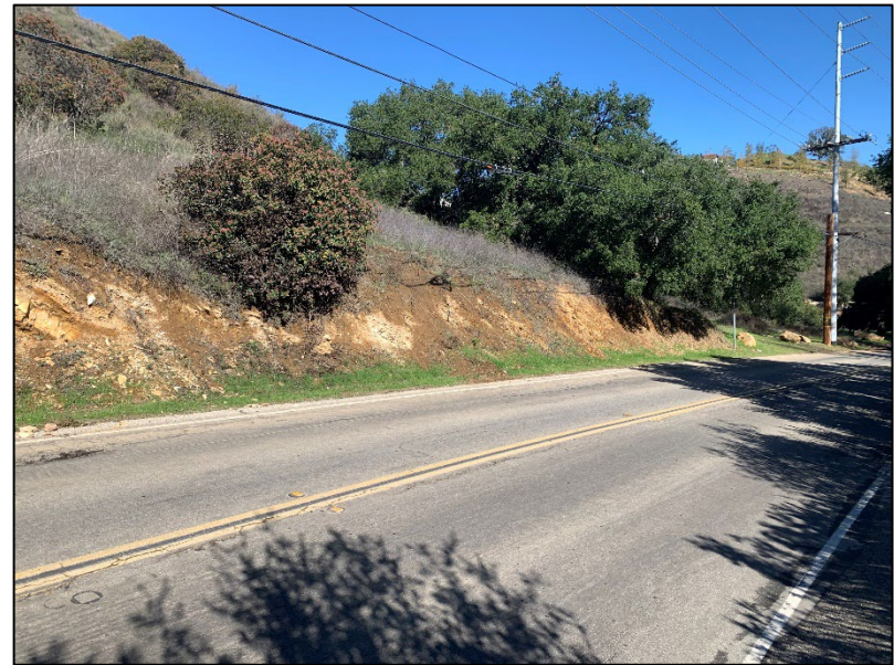
b. Slope improvement site north of Parksouth Street (STA 370)
