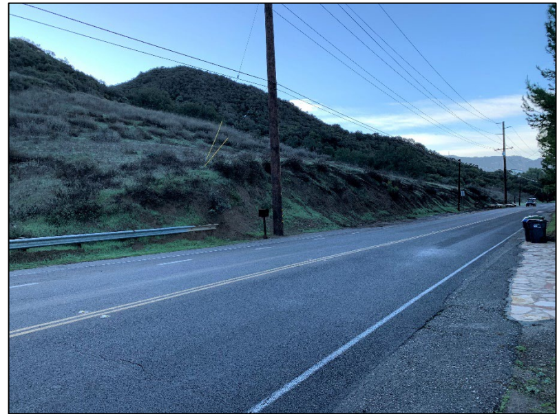
b. Slope improvement site north of Turtle Creek Road (STA 296)
