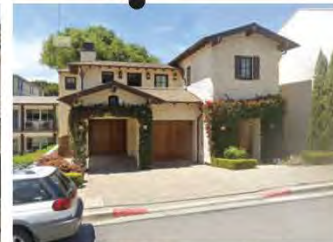
Brigantino Apartments - Rehabilitation of existing residential units.
