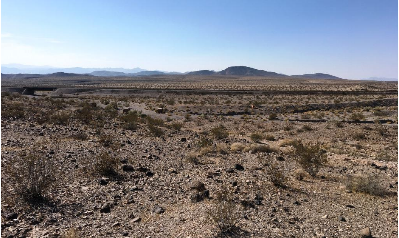
Photo 5. Looking southwest at impassable, severely eroded access route dropping into Drainage 3b north of the railroad.
