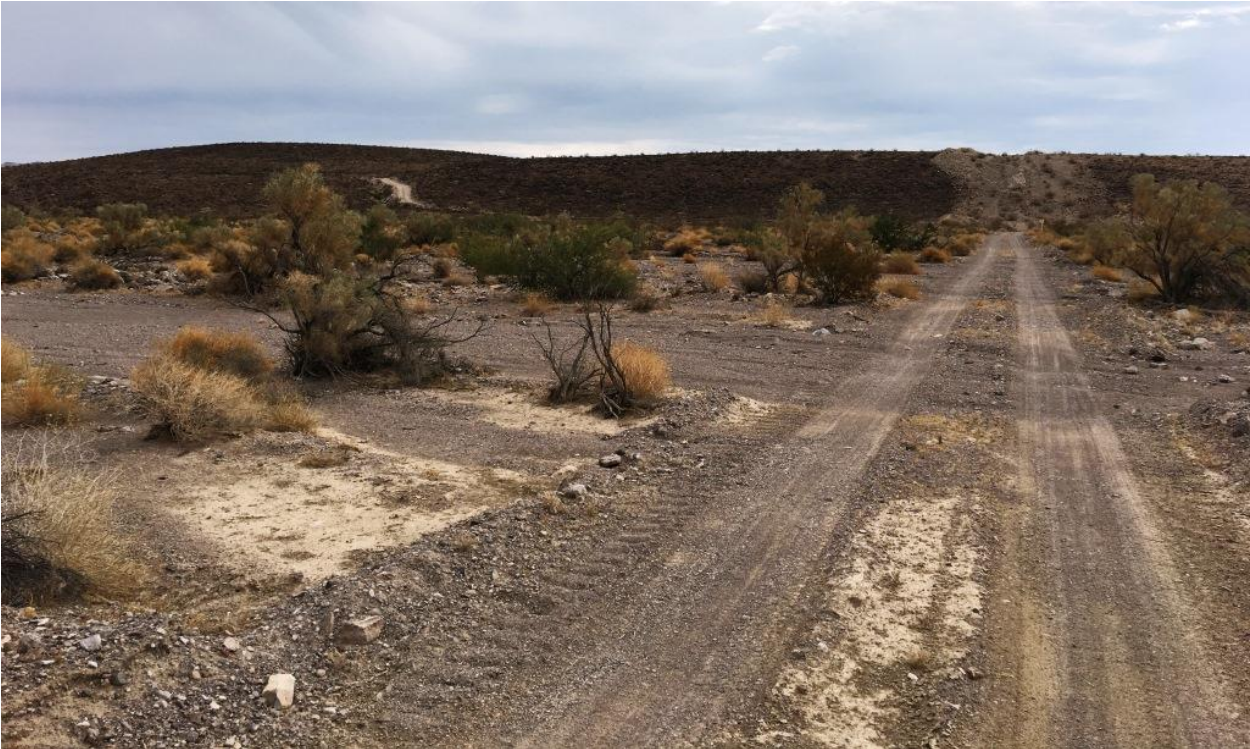
Photo 2. Typical wash conditions along the east-west gas pipeline road/NS0003.
