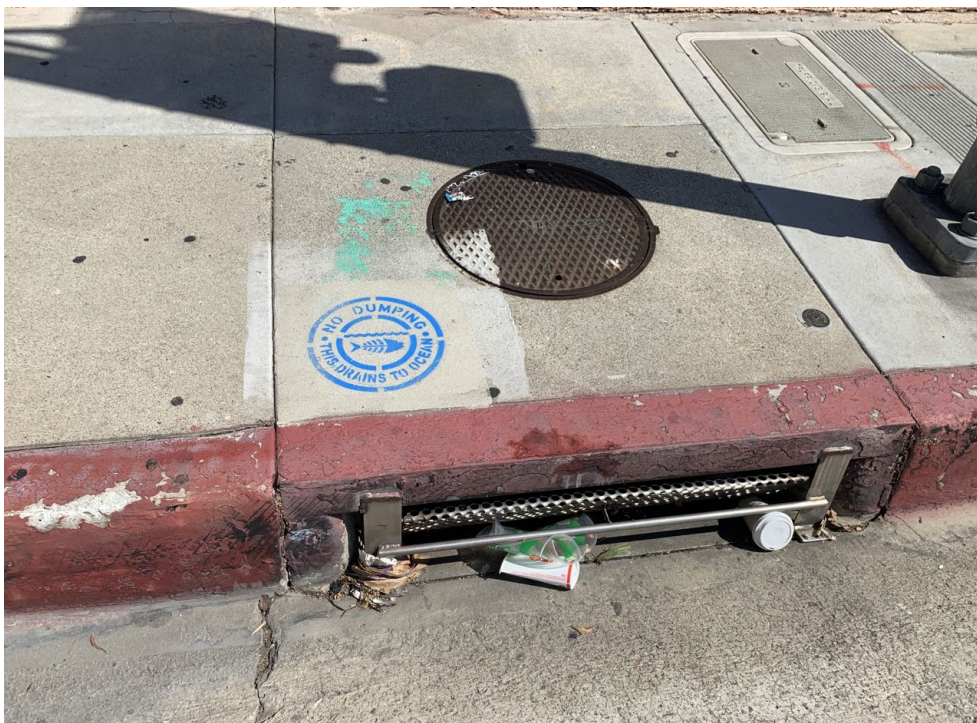
Storm drain at 58 th Street and Atlantic Boulevard that flows to ocean.
