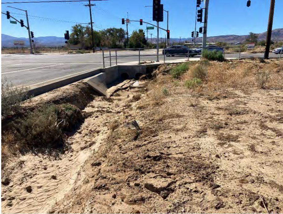
Photo 3. View of drainage southeast of the Project footprint; facing south. Drainage directs flows north to the existing natural earthen channel near the intersection of Avenue O-12 and 10 th Street East. Taken September 2022.
