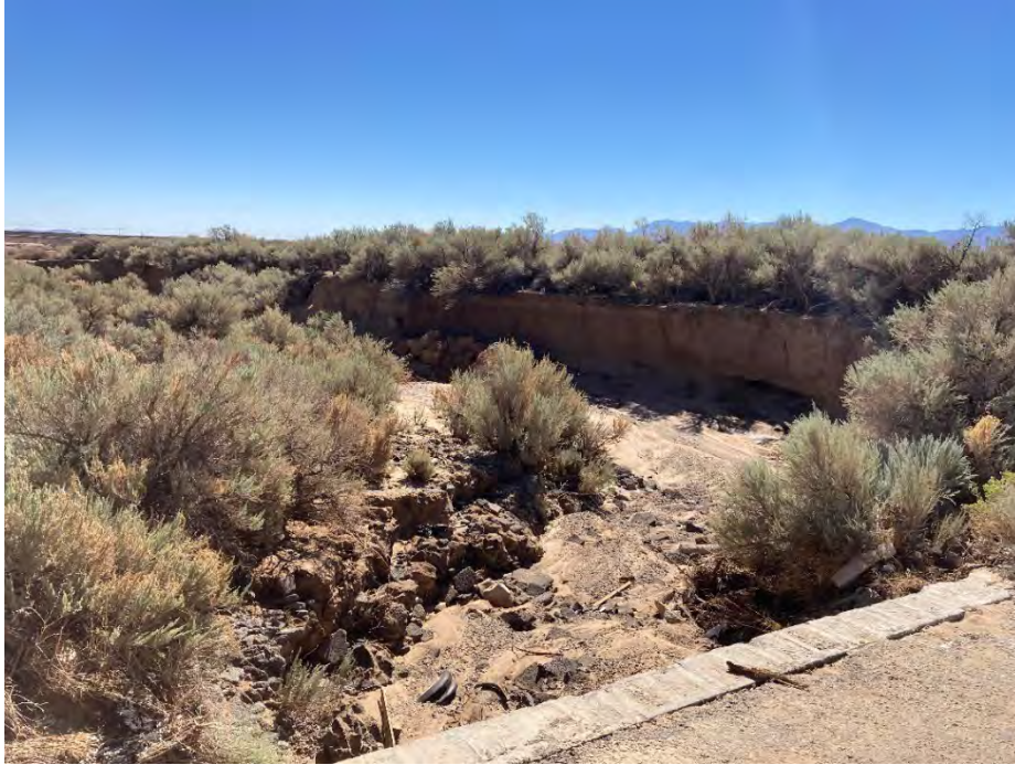
Photo 5. View of natural earthen channel located across 10 th Street East; facing east. Taken September 2022.
