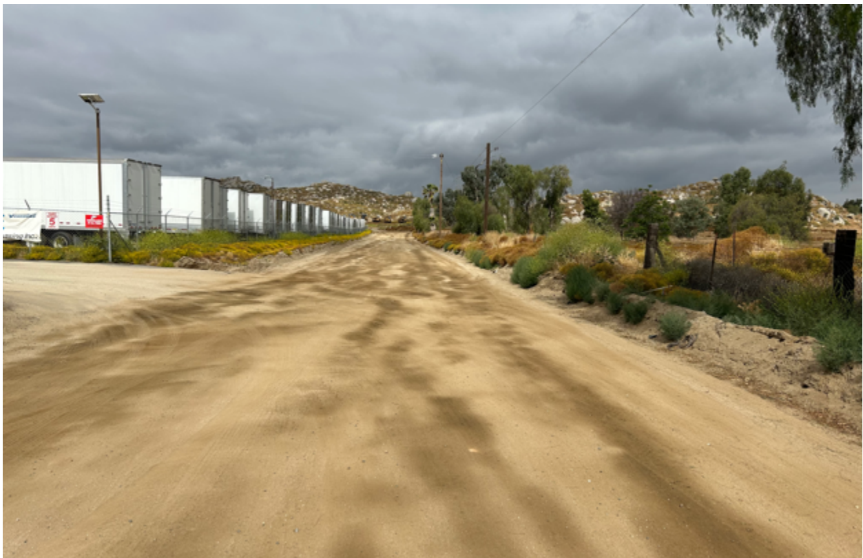
Photo 9. Approximately halfway along Water Street. Looking west toward Tobacco Road.
