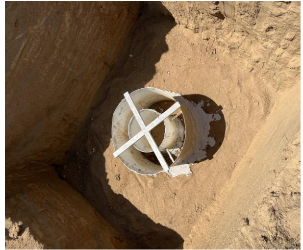
Figure 21: Using bentonite to seal the apparatus, Soil was firm and dry
