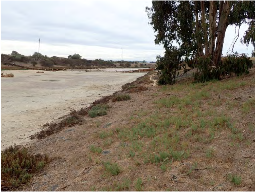
Western portion of existing WPCP basin (pond) from middle of north side. View to southwest. November 13, 2020.
