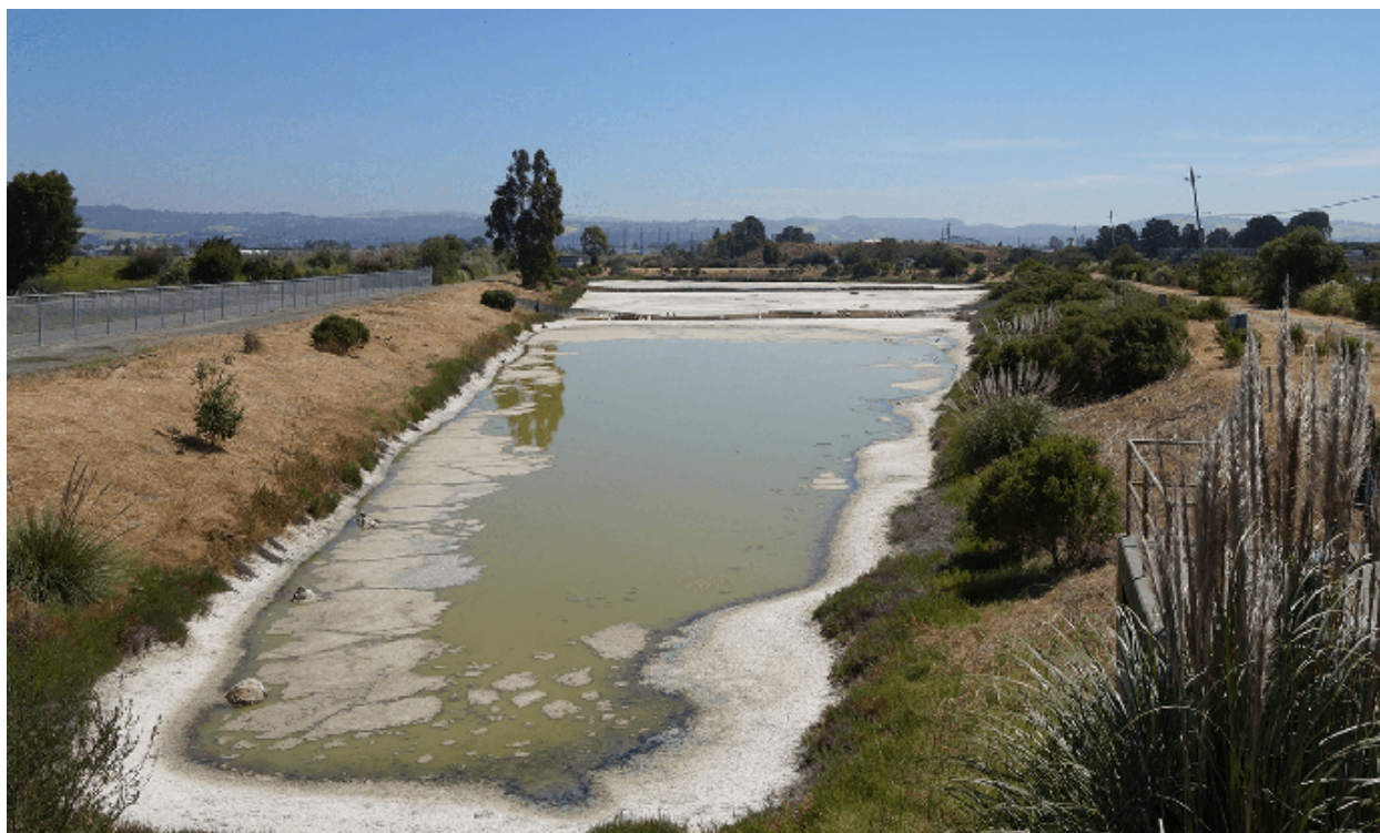
Figure 2.7. Existing conditions – east-facing view from the western edge of the existing basin
