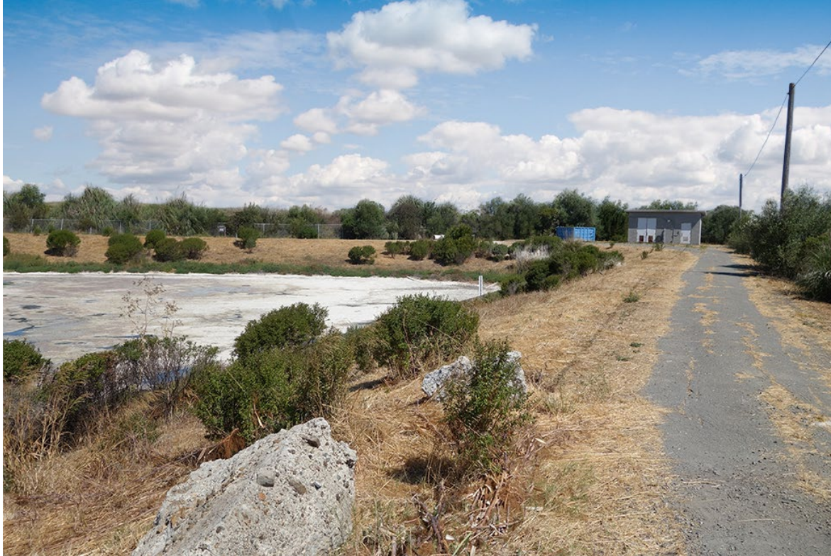
Figure 2.5. Existing conditions - east-facing view at the south-east corner of the existing retention basin
