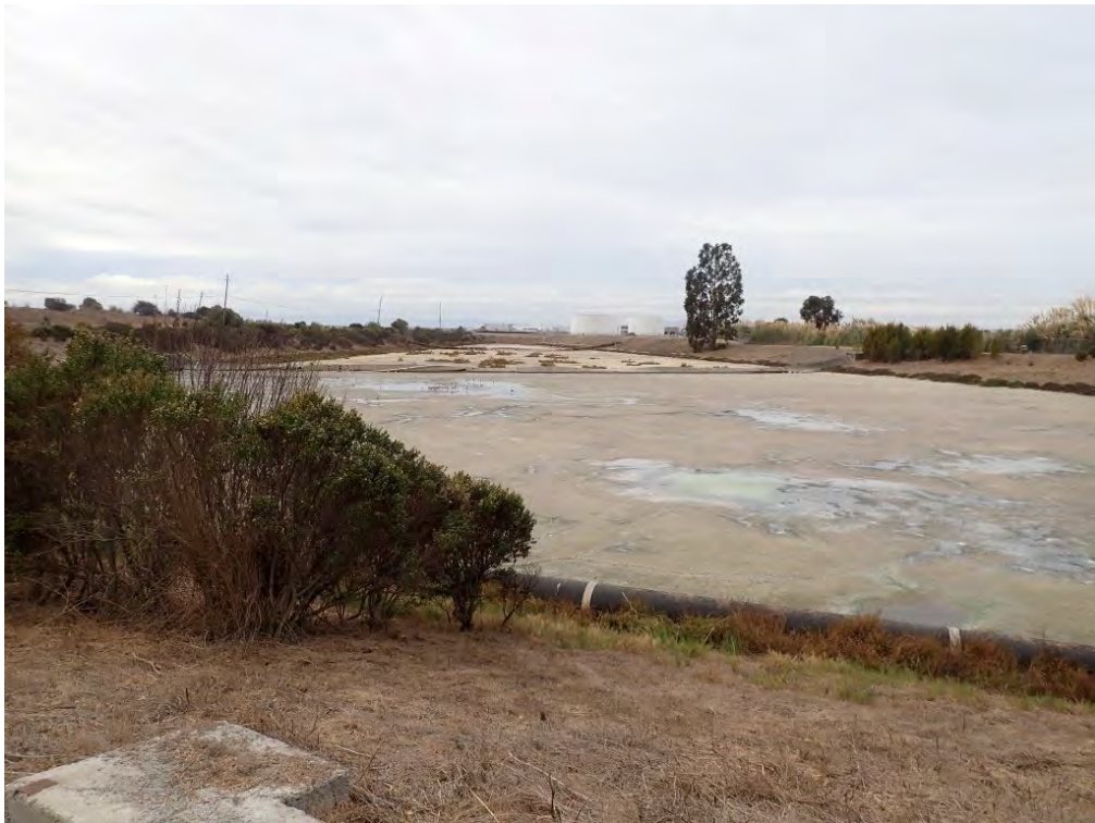
Existing WPCP basin (pond) from eastern side. View to west. November 13, 2020.
