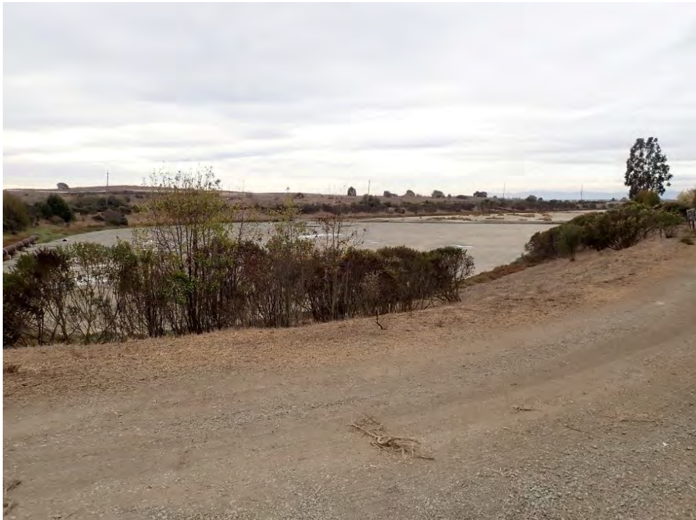
Existing WPCP basin (pond) from northeast side. View to southwest. November 13, 2020.
