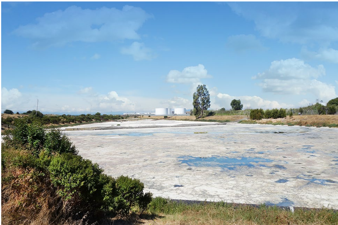
Figure 2.6. Existing conditions – west-facing view at the eastern edge of the existing retention basin
