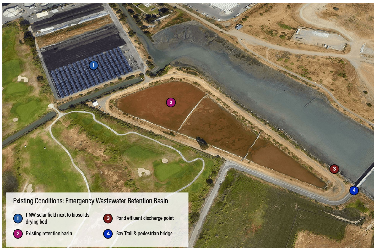
Figure 2.4. Southeast-facing aerial view of existing conditions at the Proposed Project site
