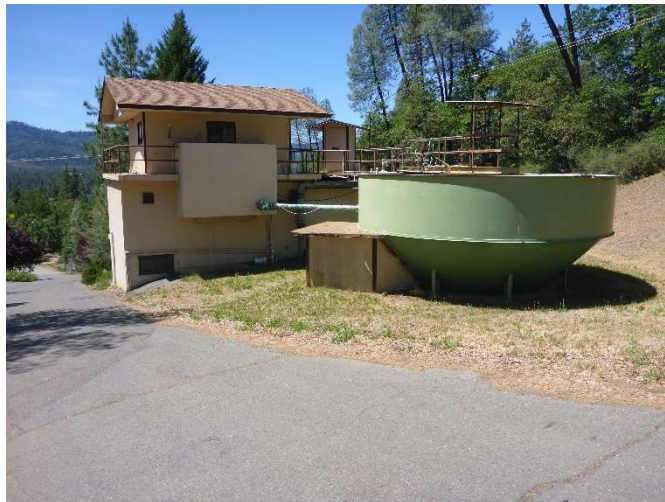
Photo 1. Existing water treatment building and clarifier
