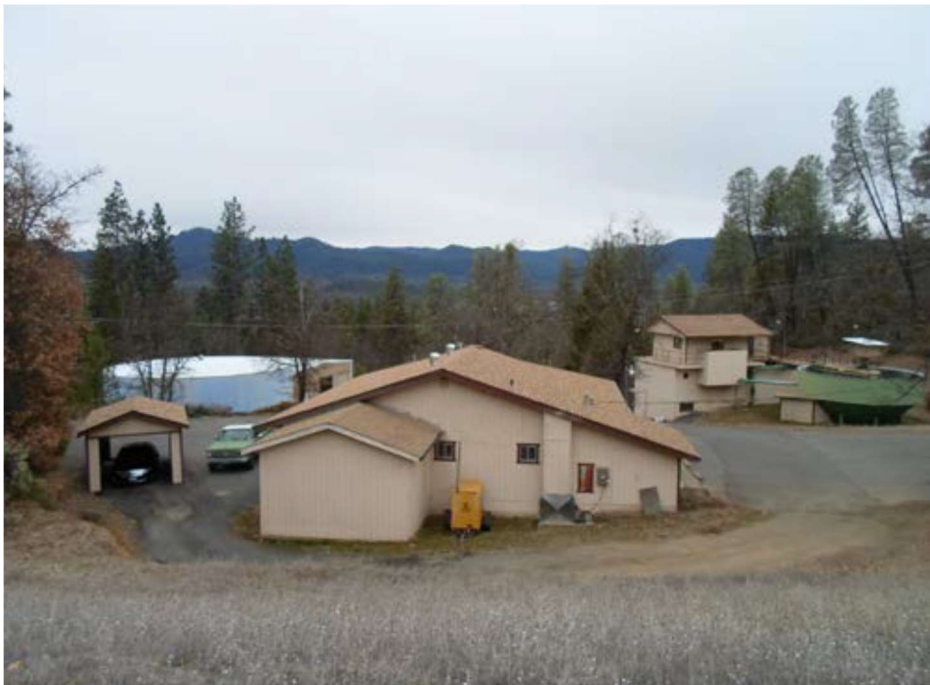
Photo 4.1-1. Existing Water Treatment Plant Facilities
