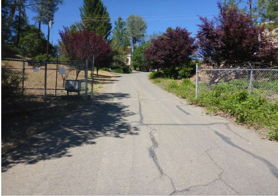
Photo 4.1-2. Entrance to Water Treatment Plant Facilities
