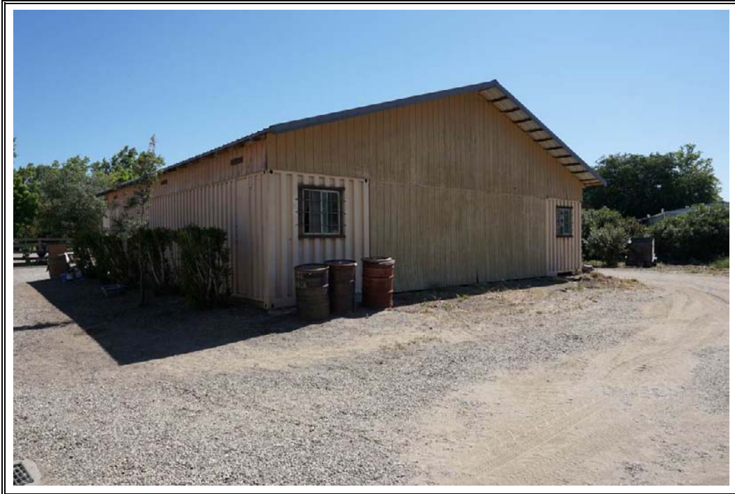
Photograph Number 13: View of maintenance shop on northeastern portion of subject property, facing east.
