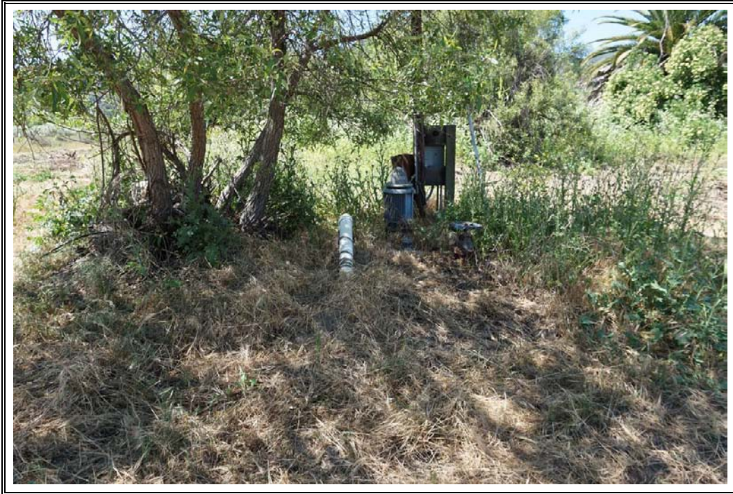
Photograph Number 27: View of irrigation groundwater well located on southern corner of subject property.
