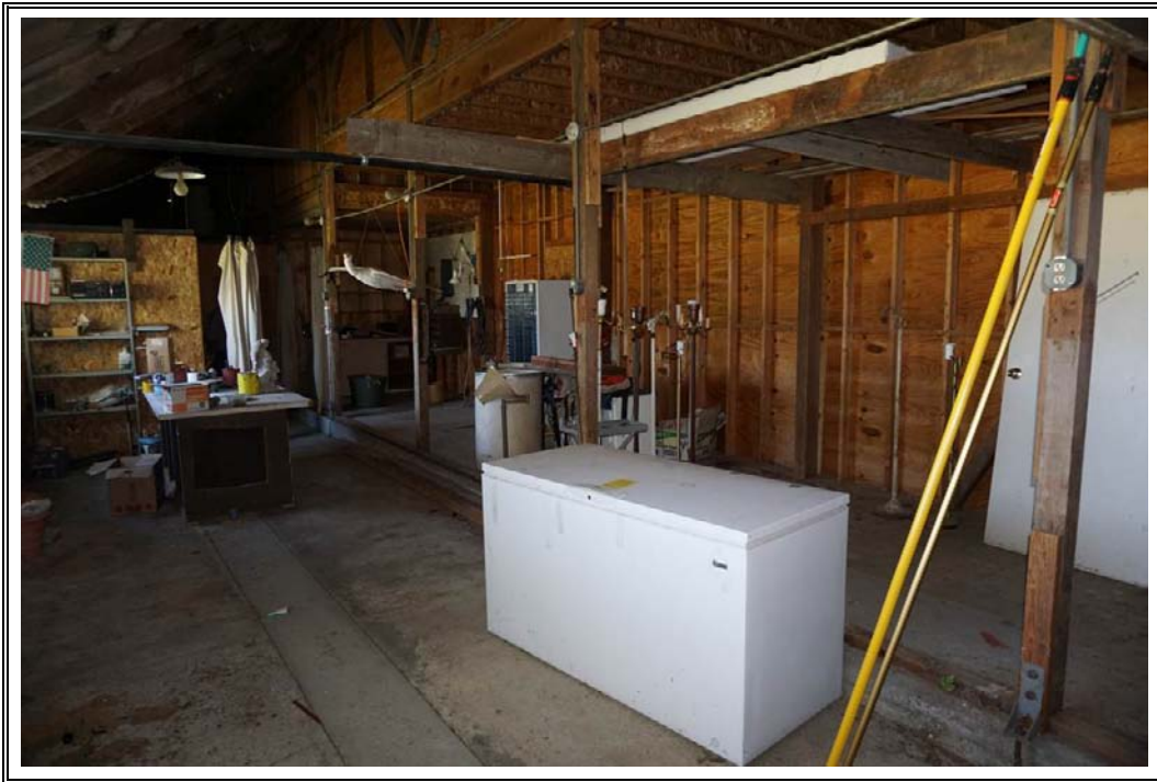
Photograph Number 37: View of barn interior.
