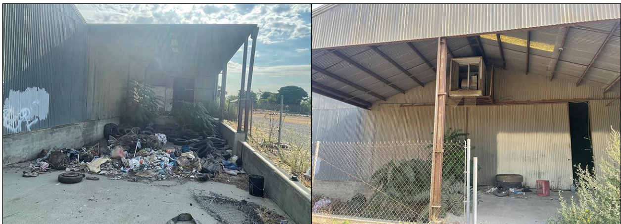
Rear and east sides, view to the southwest
