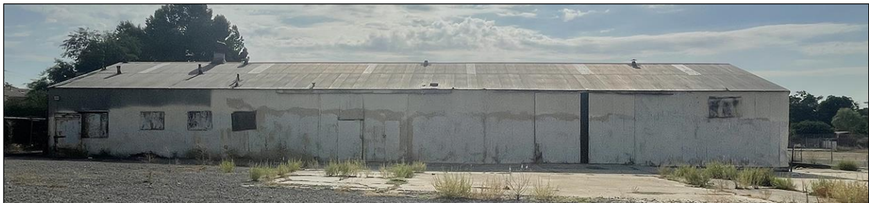
West side, view to the east
