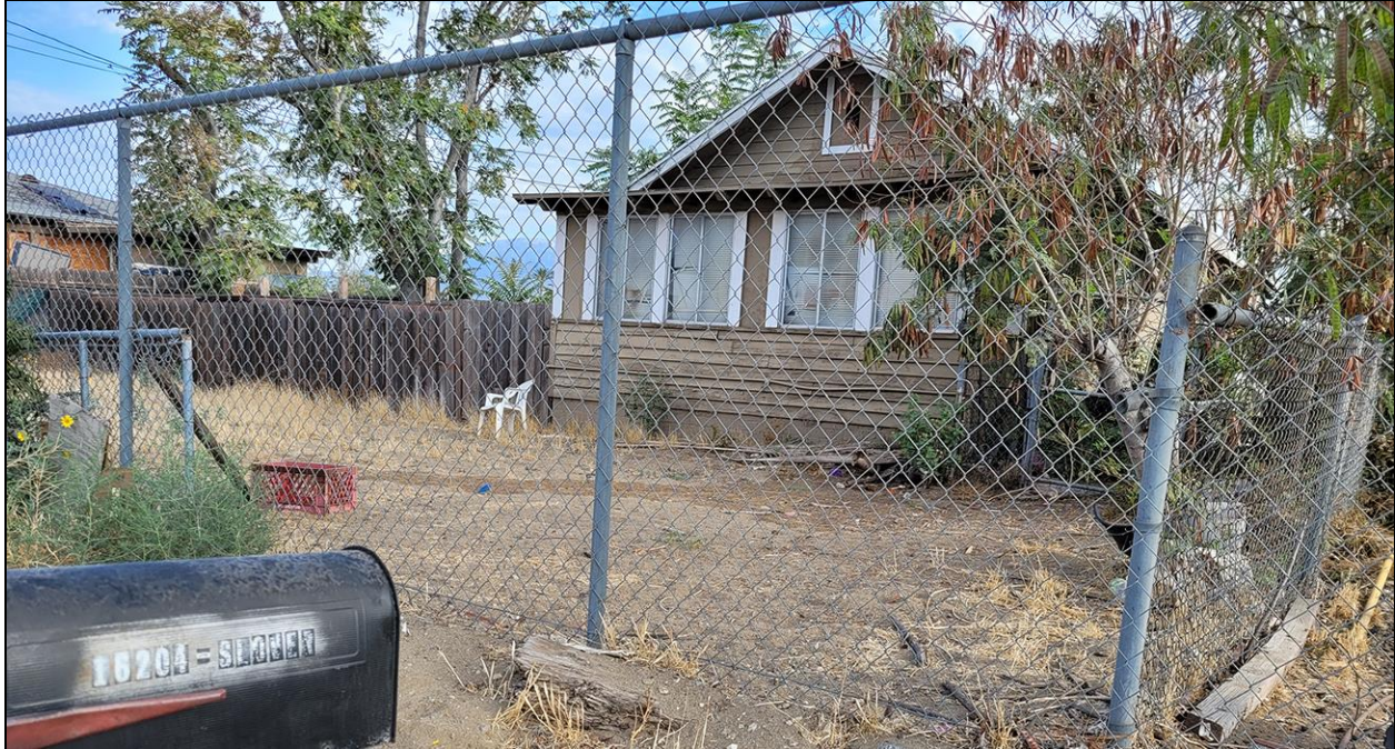
South-facing façade of the residence, view to the northwest
