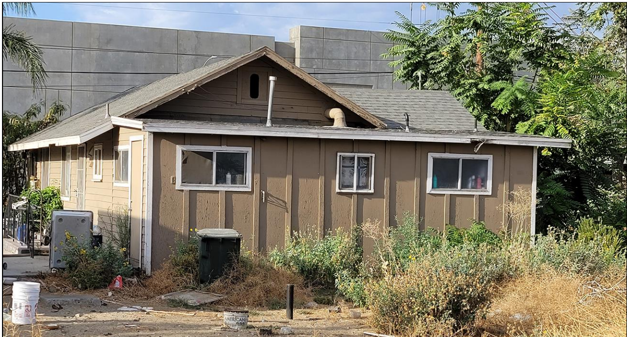
Rear and east side of the residence, view to the southwest
