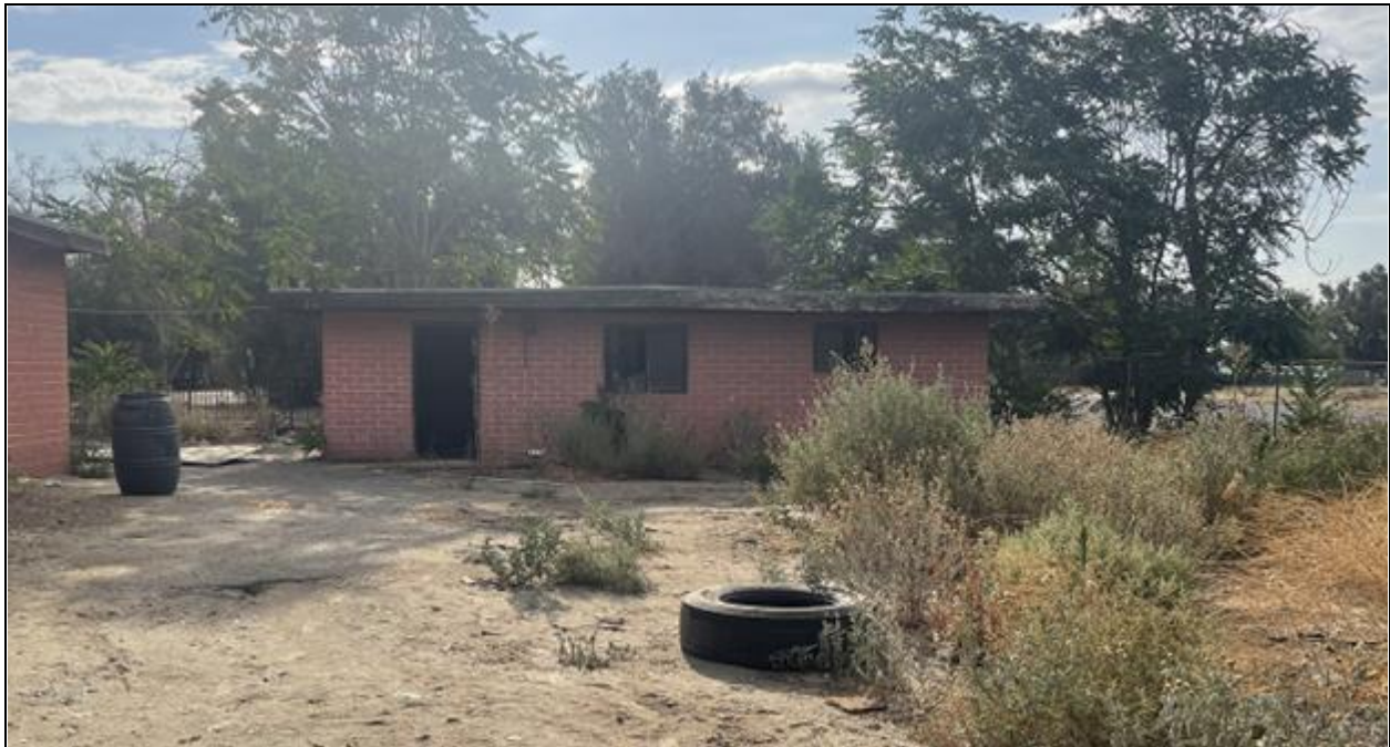
West side of the converted garage (view to the east)
