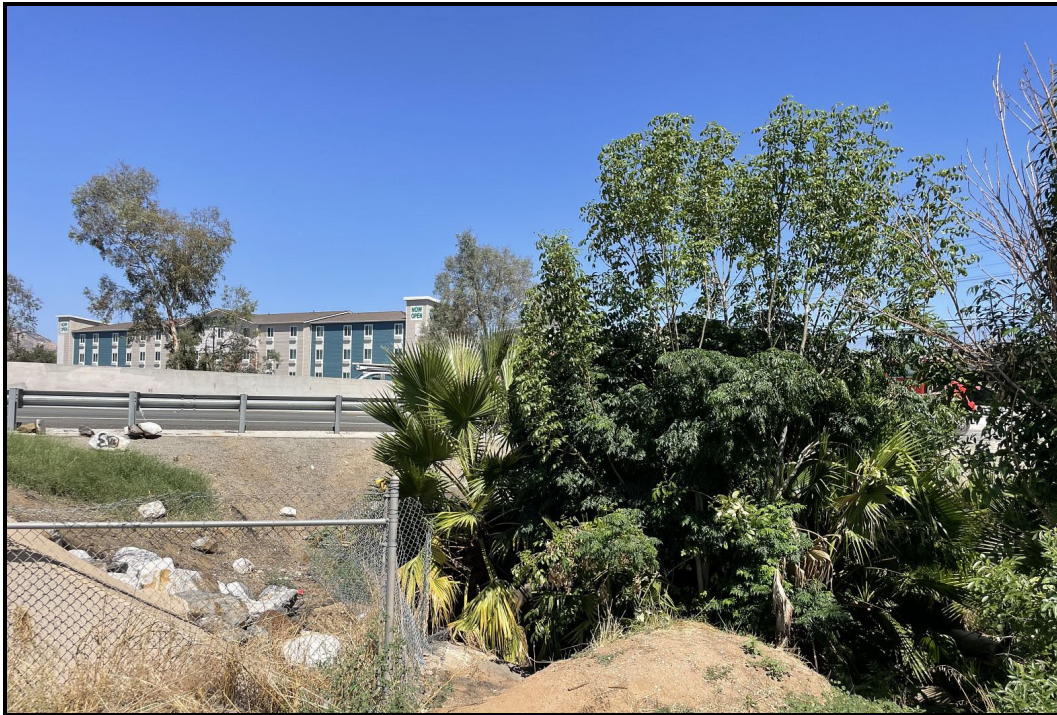
PHOTOGRAPH 5 Overview of Alignment Path Intersecting Southern Manufactured Support Slope of SR-60, Looking North-Northeast
