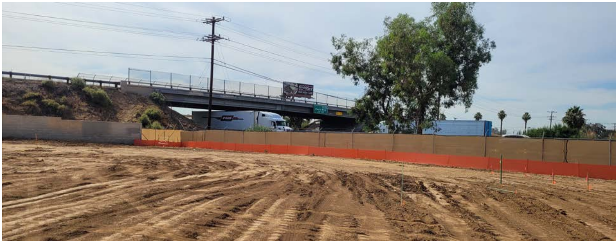
Photograph No. 4, Depicts conditions at the proposed hotel site.
