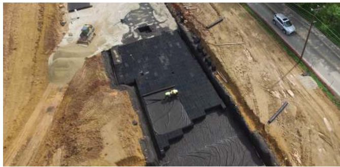
R-TANK SD INSTALLATION
