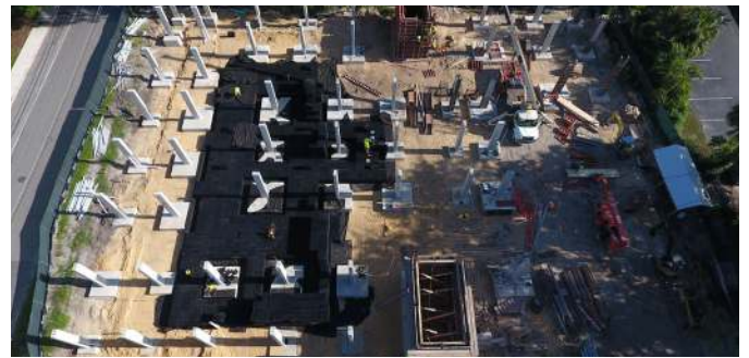
R-TANK WITHIN BUILDING FOOTPRINT
