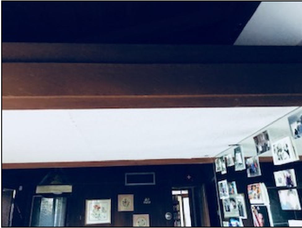
IMG_0870 - ceiling tiles between the living room and dining rooms.
