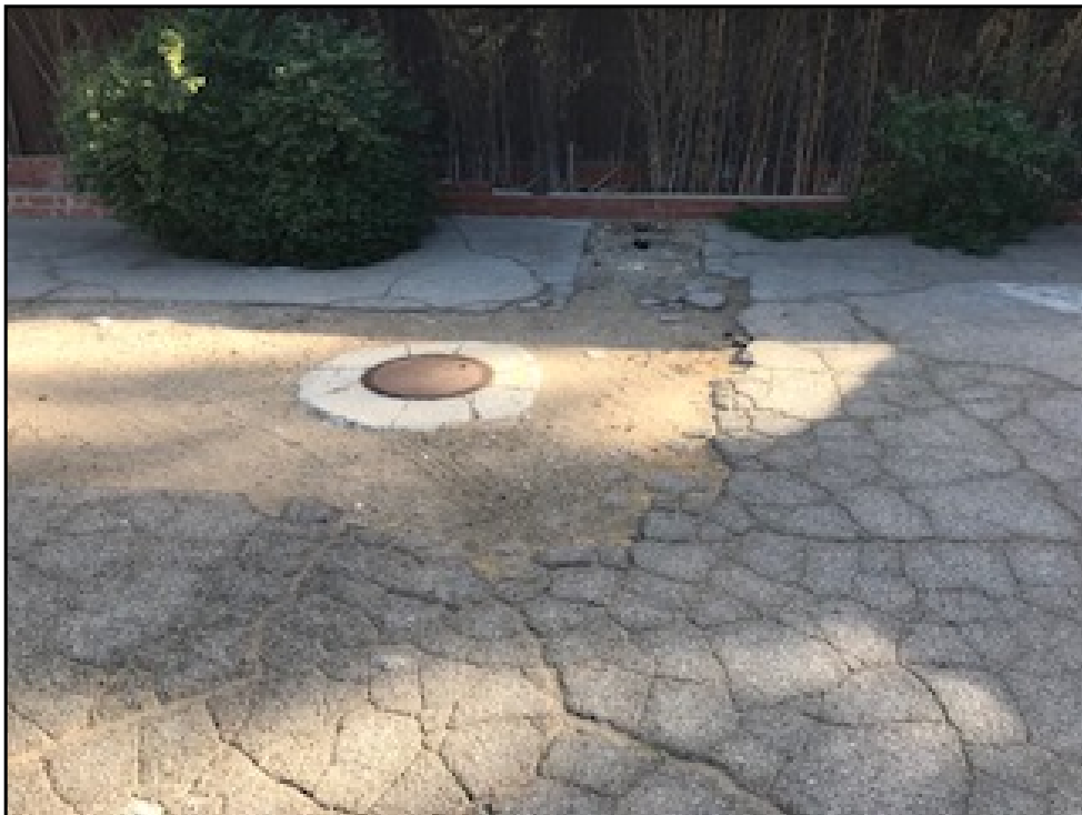
IMG_0869 - Septic tank access point out side from door in driveway.
