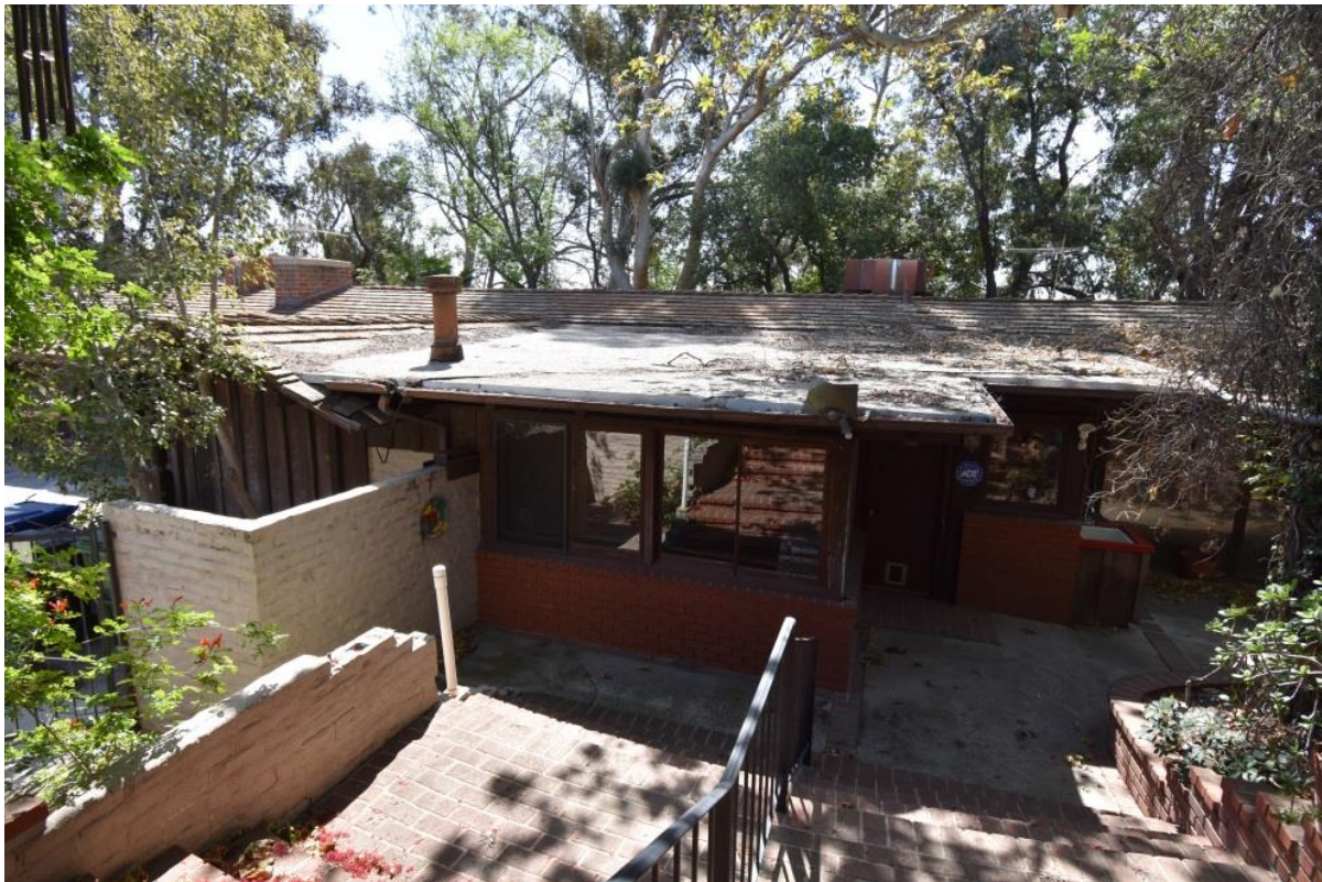
Figure 25 1973 Kitchen Addition; View to South
