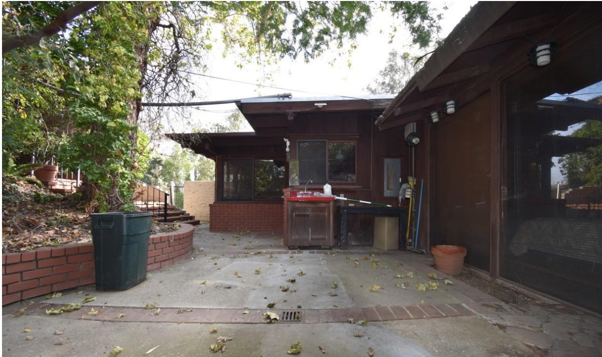
Figure 26 1973 Kitchen Addition; View to East
