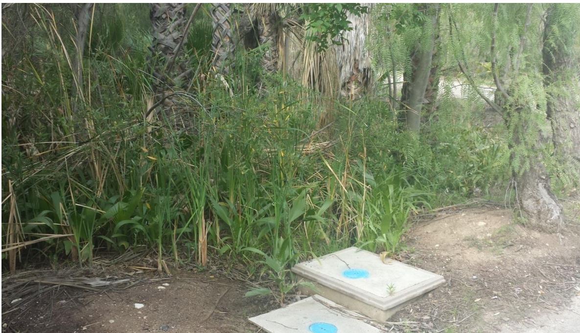
Photograph 12. View looking west at the drainage that crosses the northern portion of the project site where it is culverted under the dirt drive. Taken from the northeastern corner of the project site.
