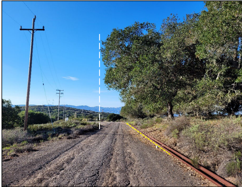
Exhibit 2. In situations where the dripline extends into the existing roadway (dashed white), as above, high-visibility flagging will be placed at the edge of the roadway (yellow).
