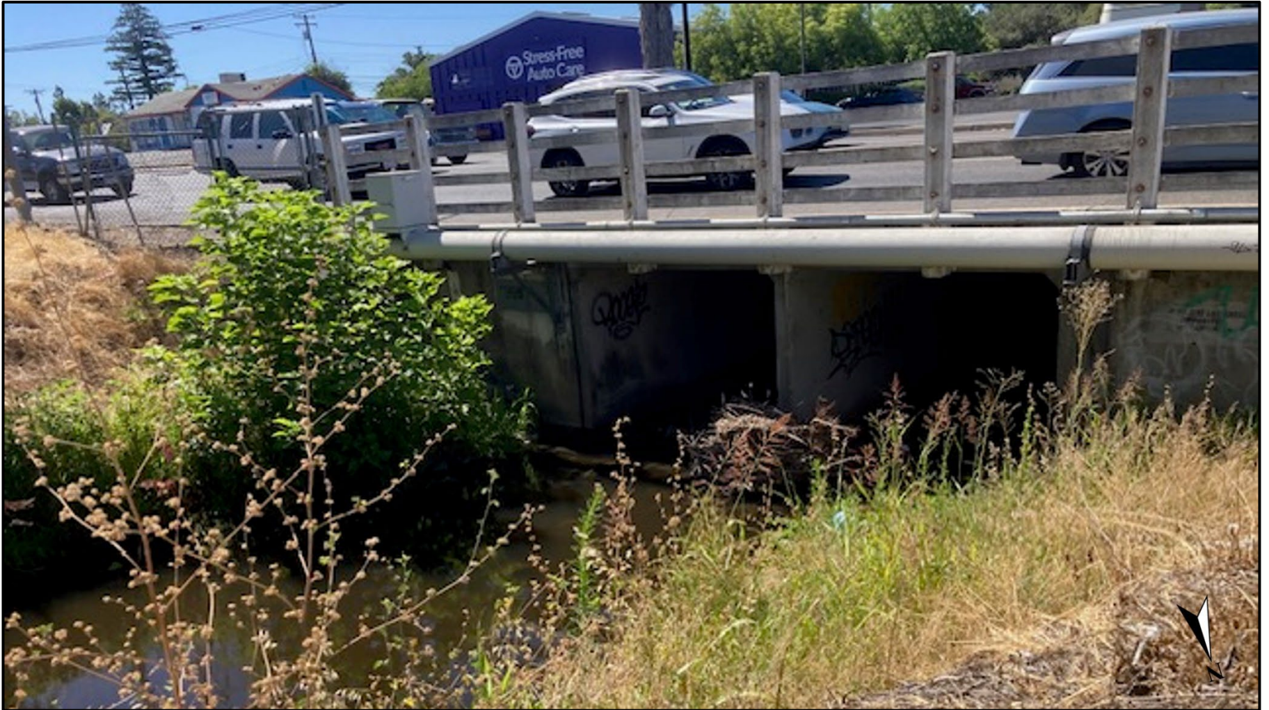
Plate IS-6: South-Facing View of Strong Ranch Slough at Arden Way
