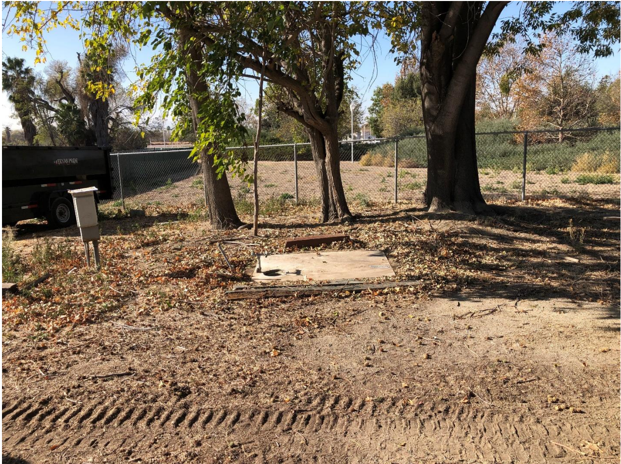
Figure 4.1-4 MAINTENANCE YARD WITH PAST WELL PLATFORM; VIEW TO THE SOUTHWEST
