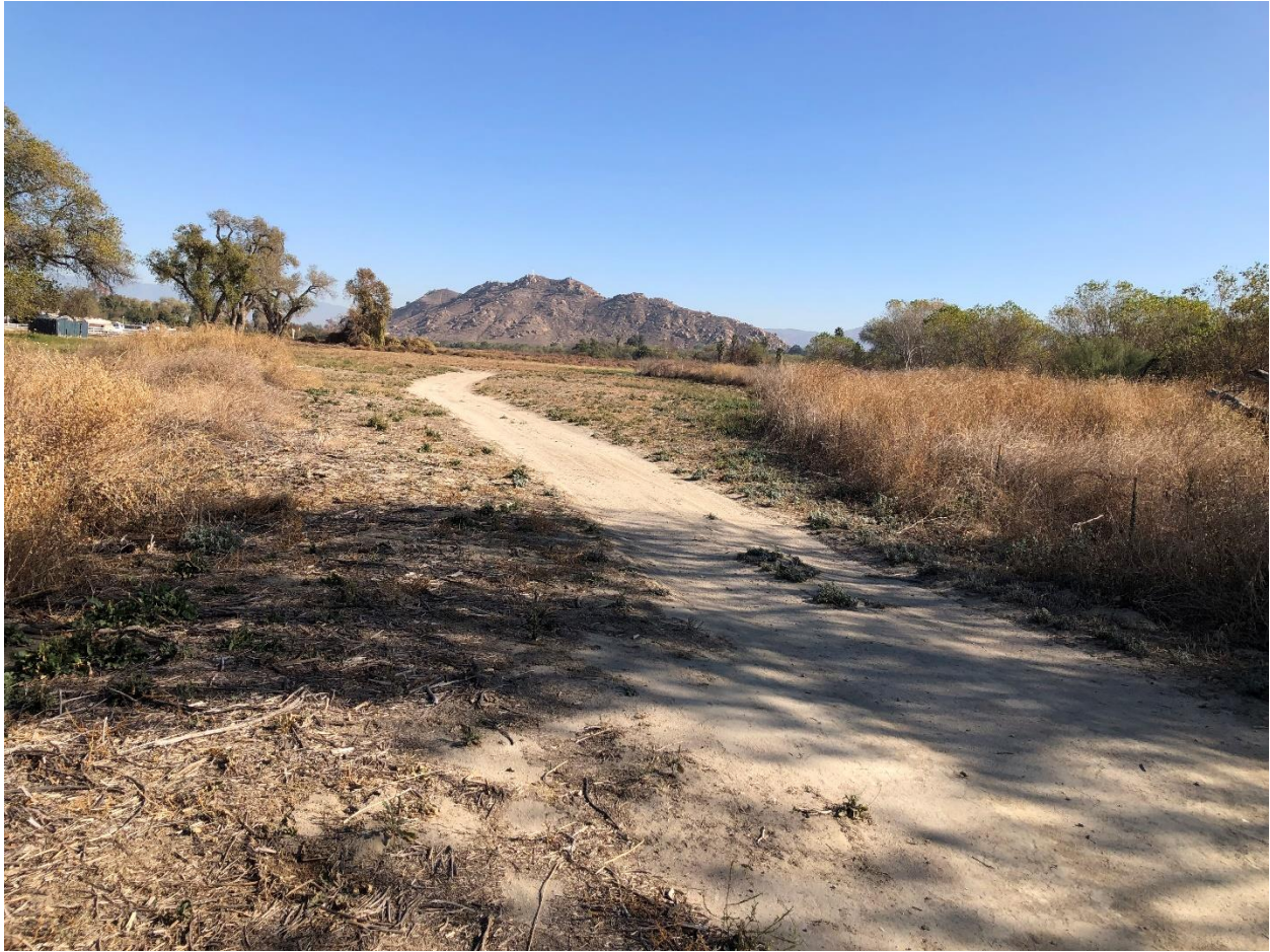
Figure 4.1-6 FENCE LINE SEGMENT ALONG SOUTH DIRT ROAD/TRAIL; VIEW TO THE NORTHEAST
