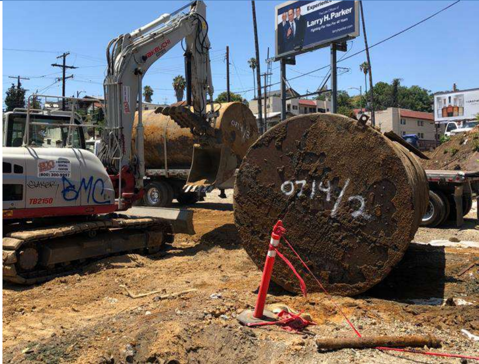
PHOTO 9: Loading the USTs in preparation for transport (07/14/22).
