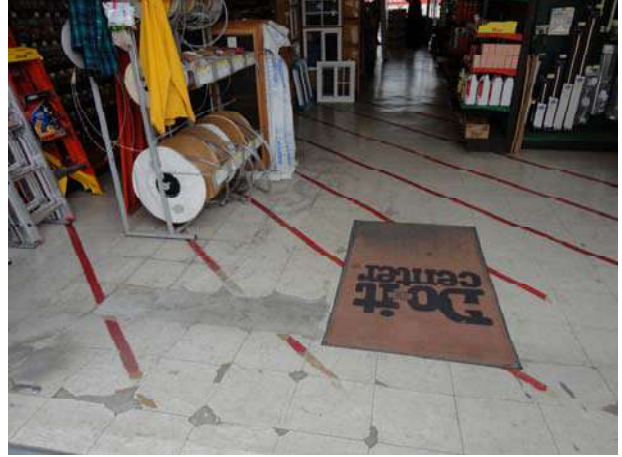
22. View of the damaged vinyl floor tiles within 1229 W. Sunset Blvd.
