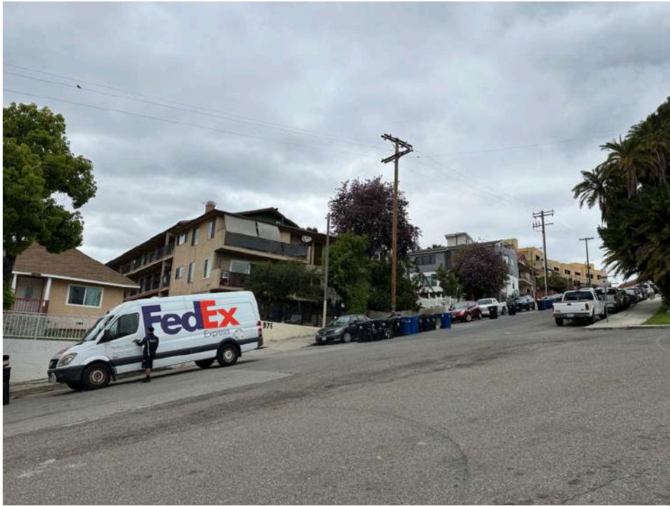
15. East adjoining residences
