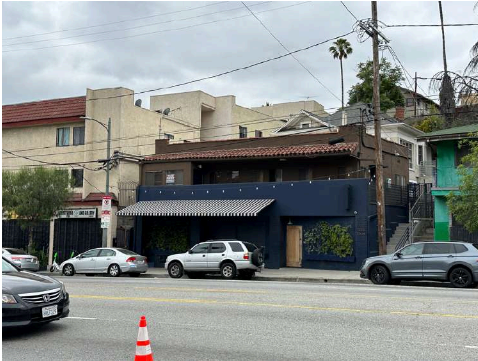
21. West adjoining mixed-use building
