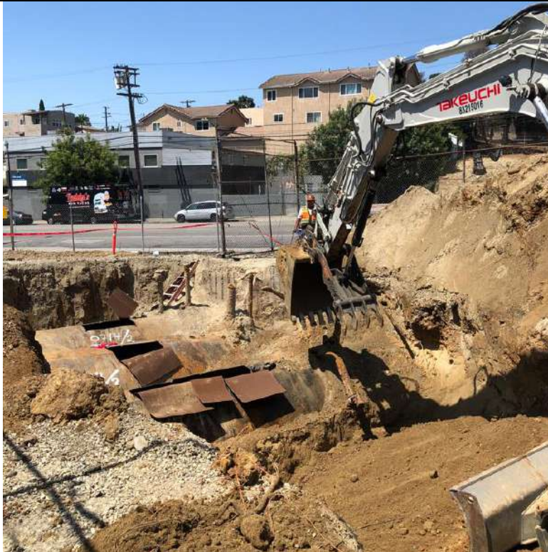
PHOTO 8: Preparing to remove the USTs (07/14/22).
