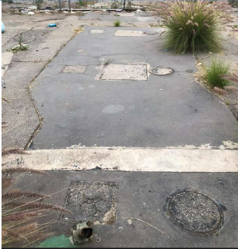
PHOTO 1: USTs prior to asphalt removal, looking south (04/28/22).
