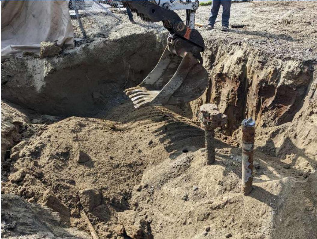
PHOTO 3: Exposing UST No. 2 (07/12/21).
