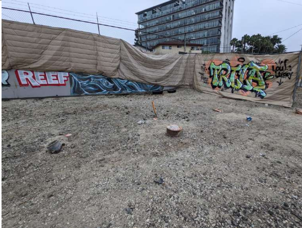
PHOTO 2: USTs after asphalt removal, looking southeast (07/12/22).
