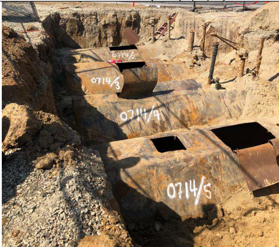
PHOTO 6: USTs certified clean and labeled, looking south (07/14/22).
