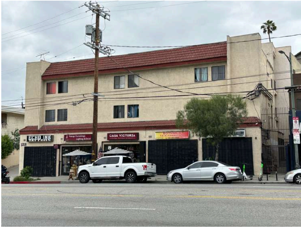
17. West adjoining mixed-use building
