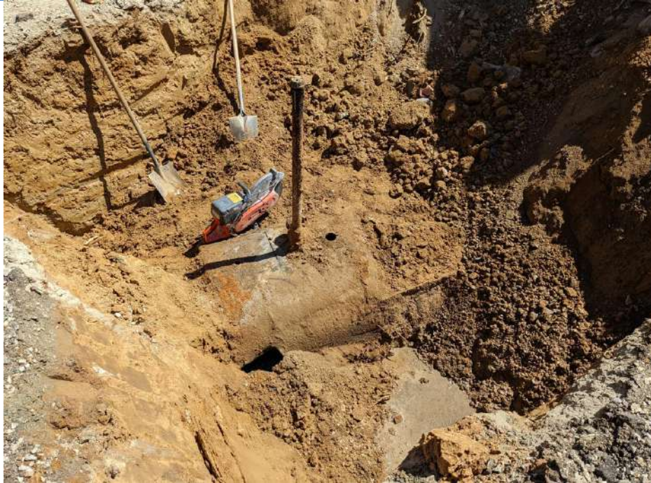
PHOTO 5: UST No. 6 exposed (07/12/22).
