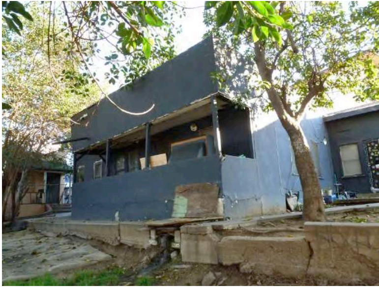
Figure 11: West façade of 1245 West Sunset Boulevard. Source: GPA.
