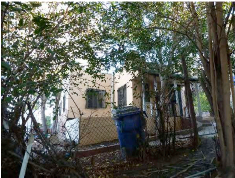
Figure 12: South façade of 1247 West Sunset Boulevard. Source: GPA.
