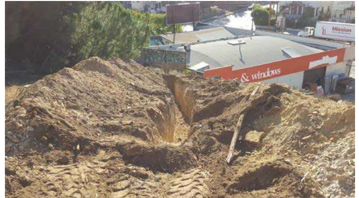
Photo 62 – Test Pit 24 General Vicinity
