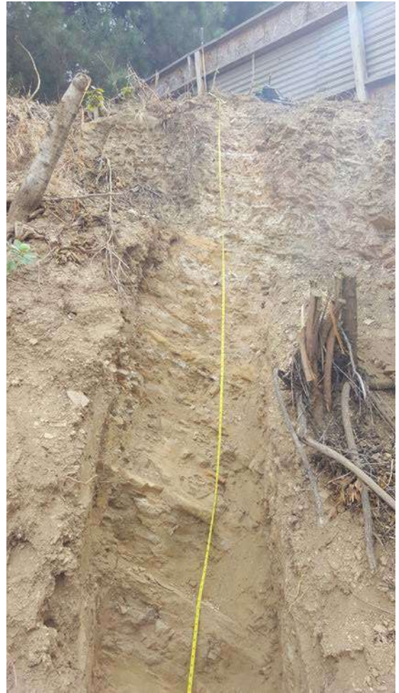
Photo 46 – Test Pit 22 A
