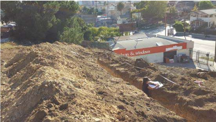
Photo 49 – Test Pit 23 General Vicinity
