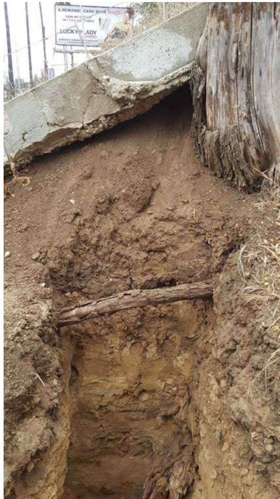
Photo 14 – Test Pit 9 A
