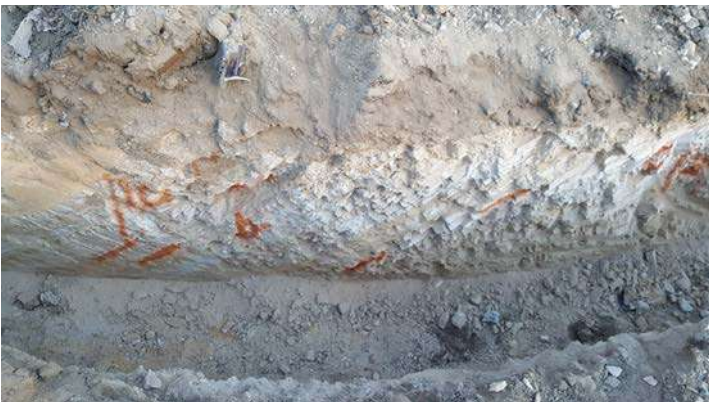
Photo 65 – Test Pit 24 C
