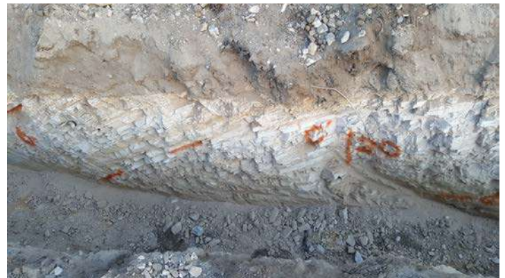
Photo 66 – Test Pit 24 D
