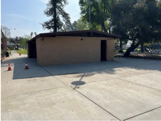
Overview of restroom building, facing east.
