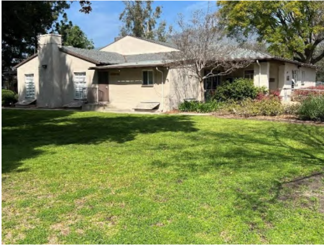
Overview of American Legion Building, facing northwest.
