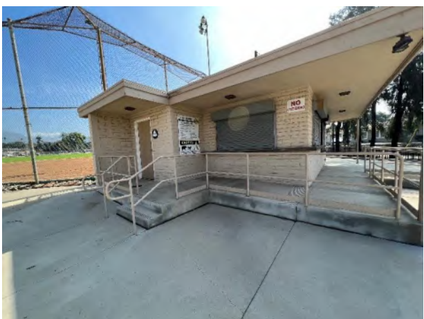
Overview of concessions and restroom building, facing northeast.
