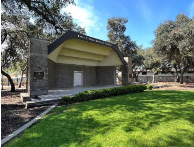
Overview of bandshell facing southwest.
