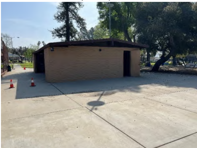
Overview of restroom building, facing east.
