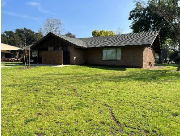
Overview of Rotary Scout Hut building, facing northeast.
