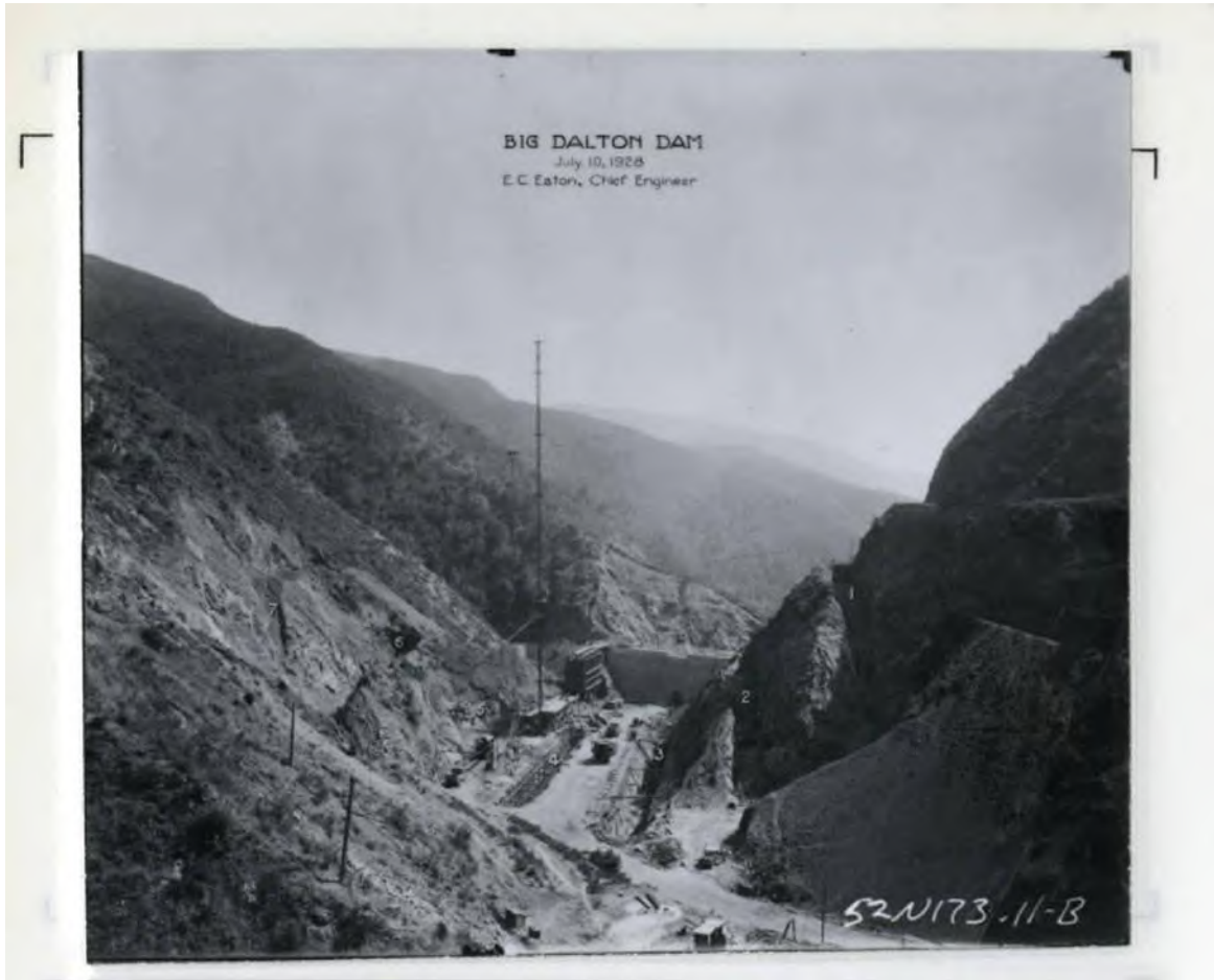
Exhibit 1. Big Dalton Dam (Los Angeles County Library 1928)
