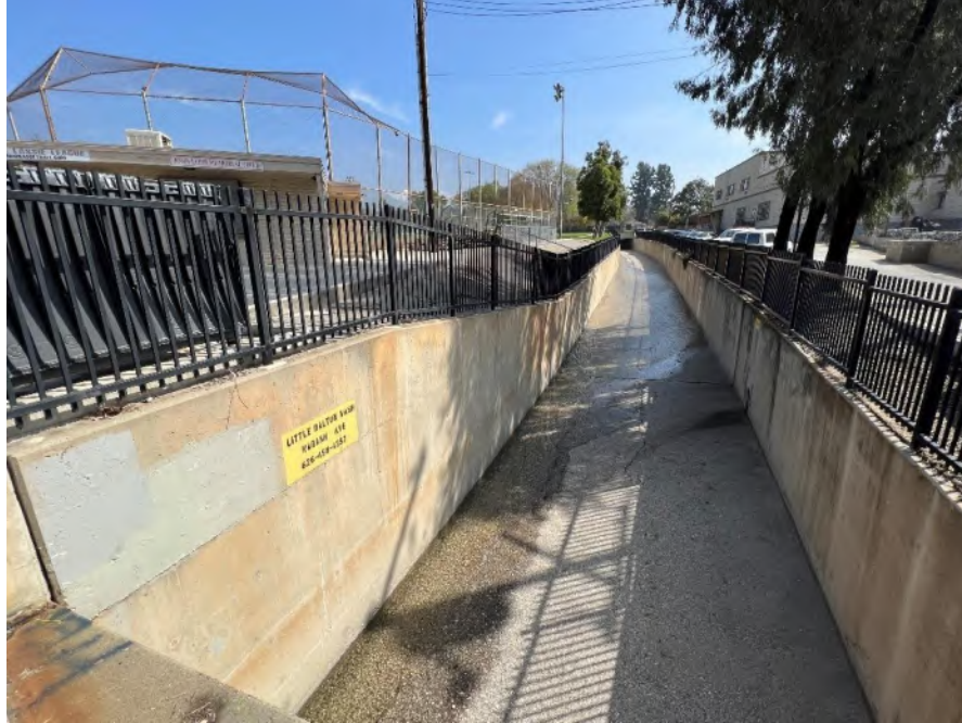
Photograph 1. Overview of Little Dalton Wash, facing northeast.
