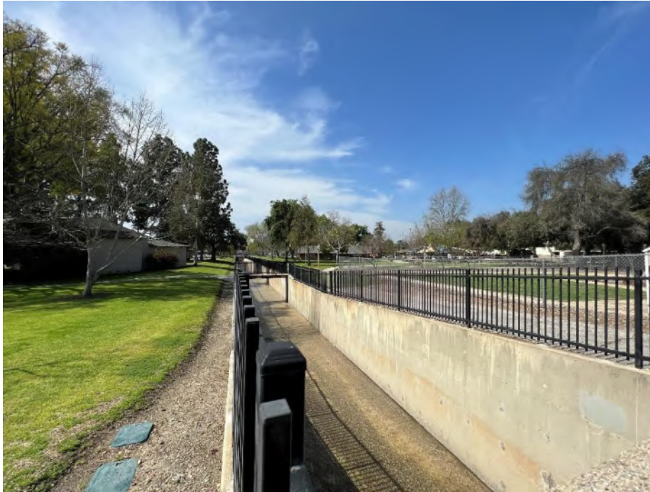
Exhibit 6. Overview of pedestrian crossing north of American Legion Building, facing southwest.
