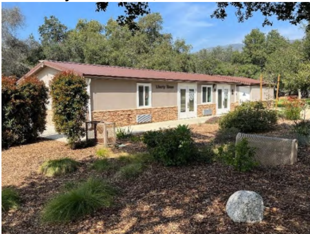
Overview of Liberty House, facing northwest.
