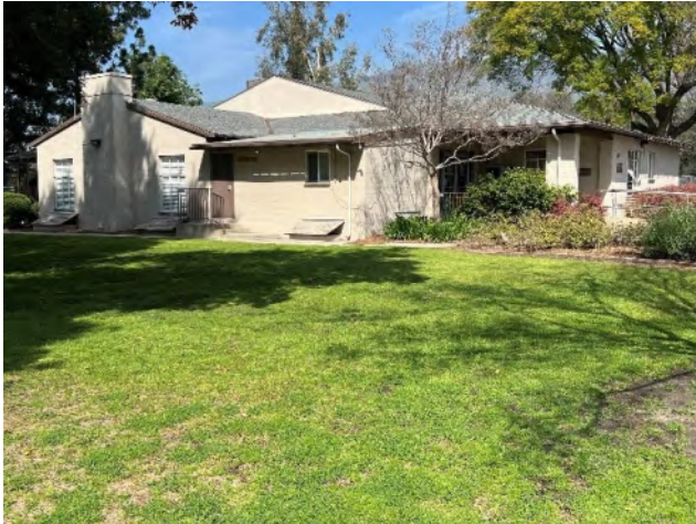
Overview of American Legion Building, facing northwest.
