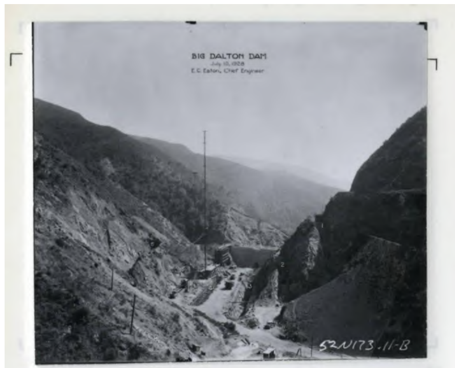
Exhibit 1. Big Dalton Dam (Los Angeles County Library 1928)
