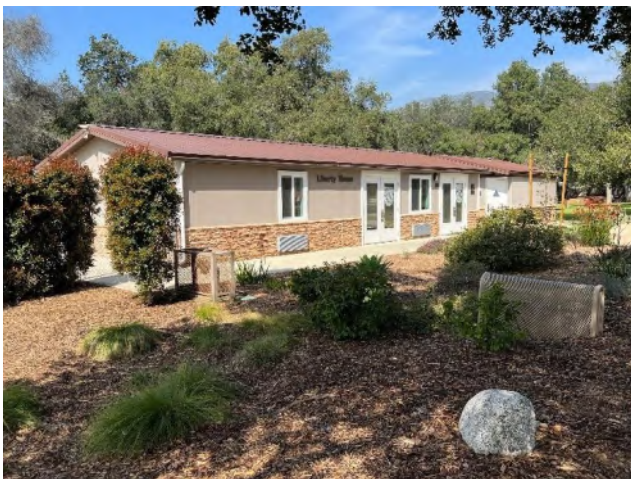
Overview of Liberty House, facing northwest.
