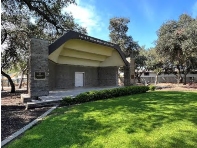
Overview of bandshell facing southwest.
