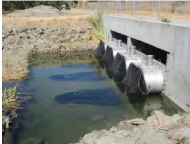
Representative Image 4. Example of End-of-Pipe Netting System
