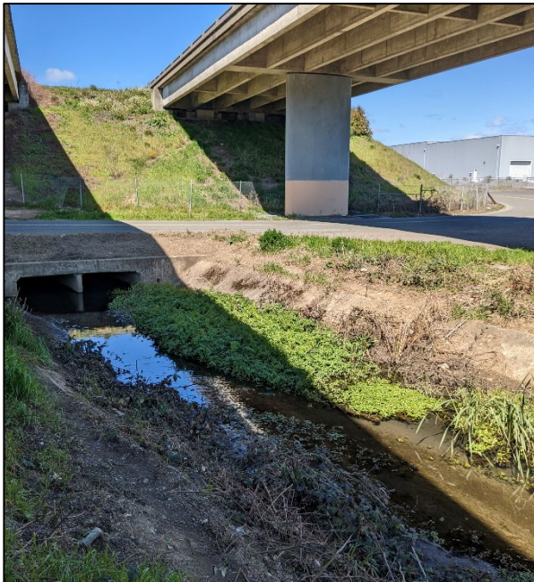
Photo 7. Cemented box culvert at UK.21 (April 4, 2023).
