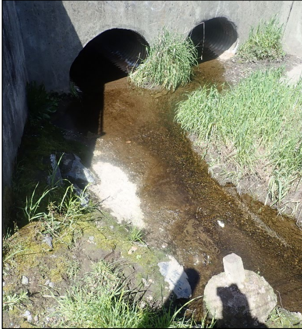
Photo 1. Intermittent stream and wingwall at UK.10 (April 4, 2023).
