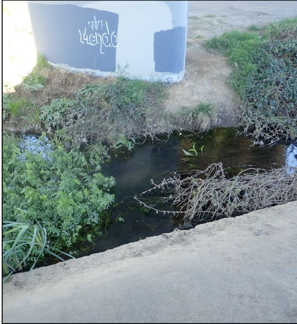
Photo 9. Intermittent stream at UK.22. The eastern slope is concrete lined (April 4, 2023).
