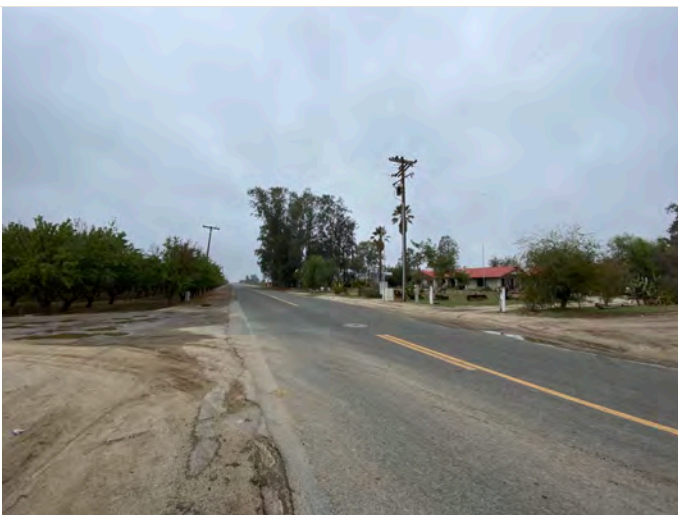
view west to alignment shift to avoid settlement
