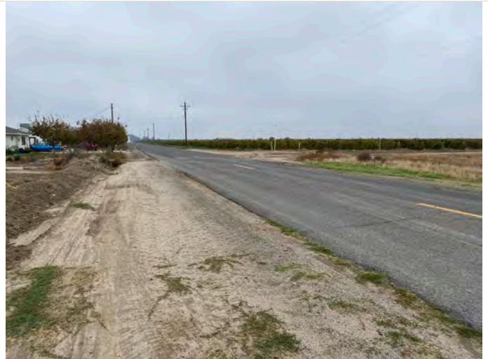
view west; Jensen crossing for east side canal
