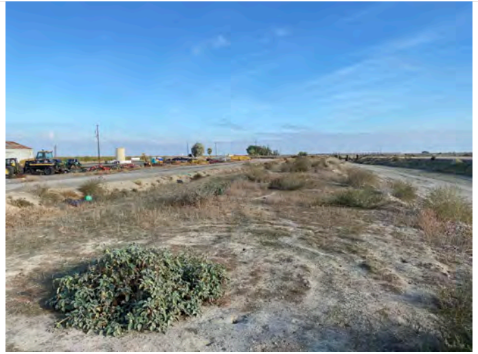
view east towards S. James Rd and pump station locations from top of canal
