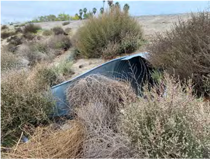
view NW culvert under CA 180
