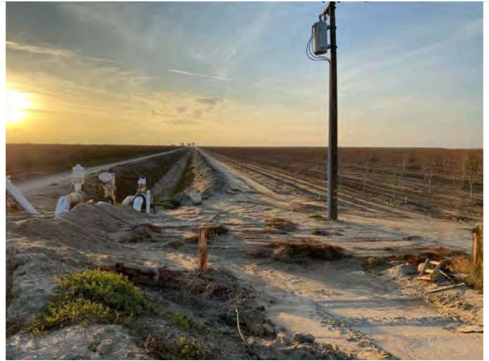
view west canal and pump infrastructure
