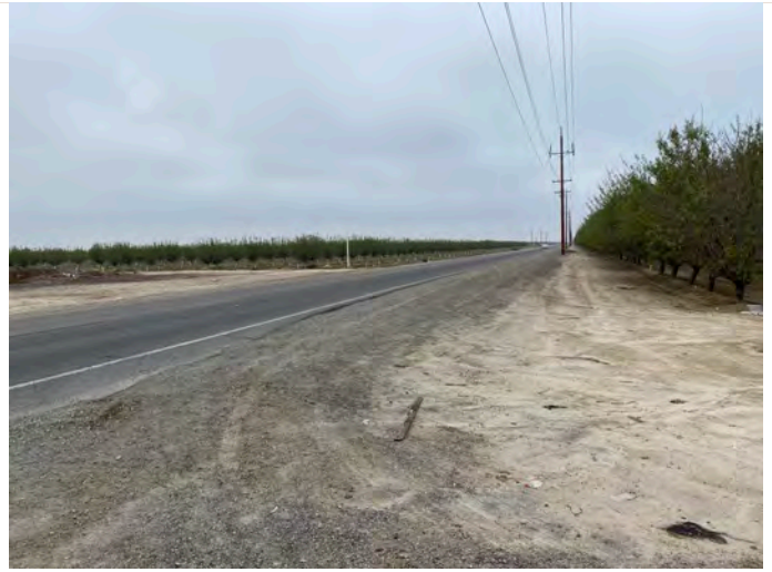
view west down James Alignment and at pump station location proposed
