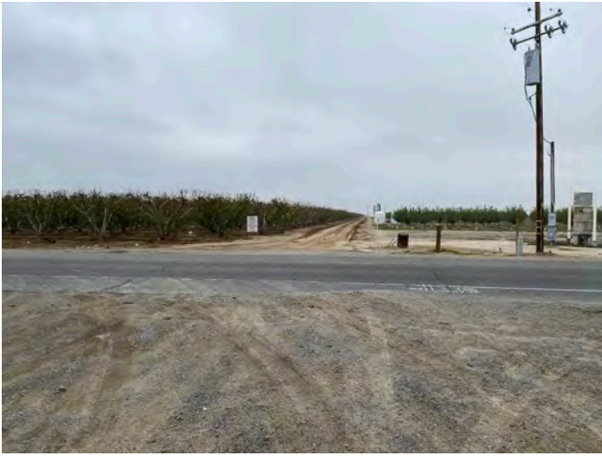
view south down Siskiyou Canal
