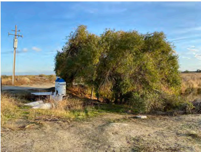
View east at pump station location
