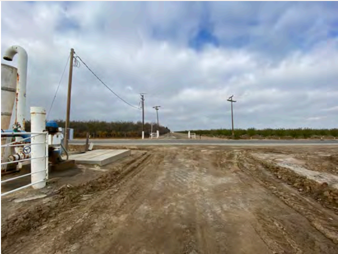
view north at canal alignment crossing at Manning Avenue
