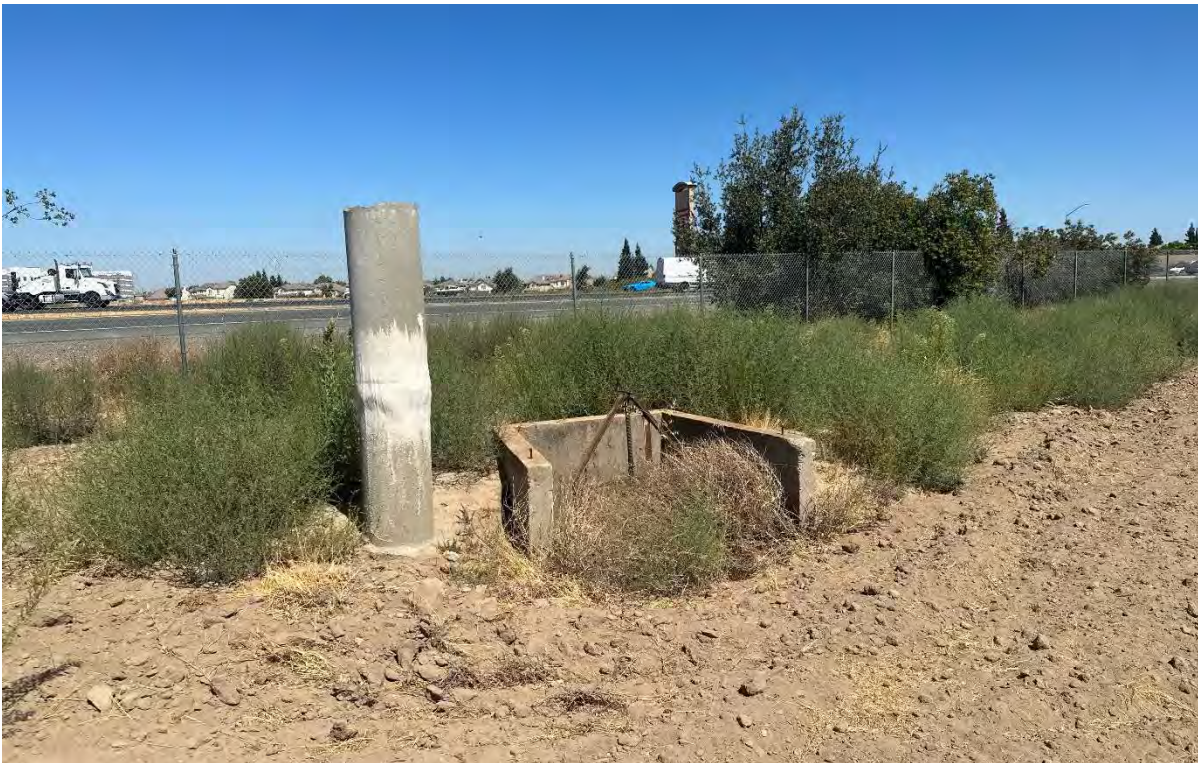
Photograph 4 Overview of Water Conveyance Feature, View to the North
