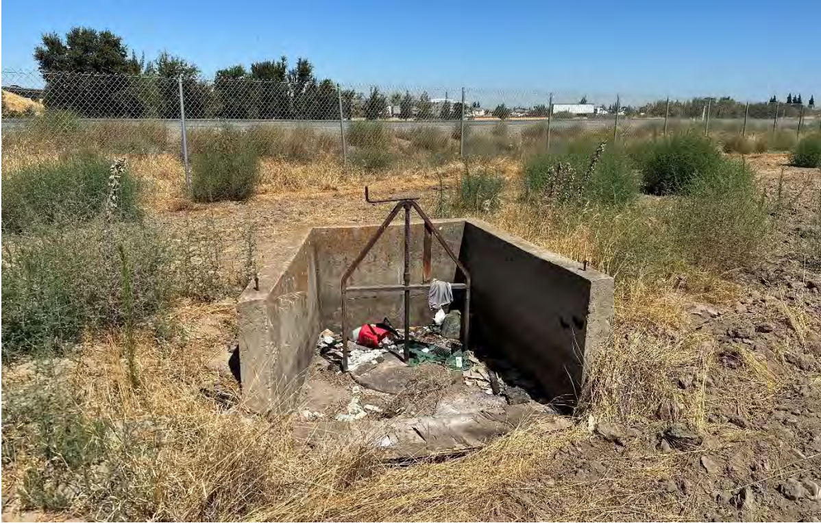
Photograph 3 Overview of Water Conveyance Feature, View to the North
